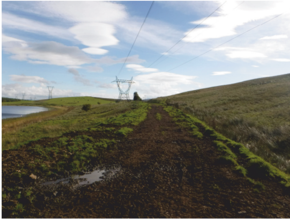
Fig. 5 - General view over Site D - Railway, looking north
