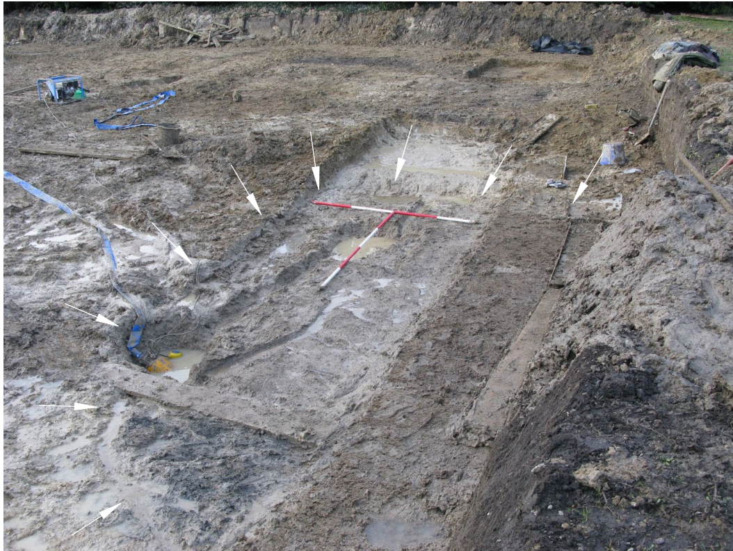
Fig. 7 - Shot of feature 292 prior to machine excavation, taken from the SE
