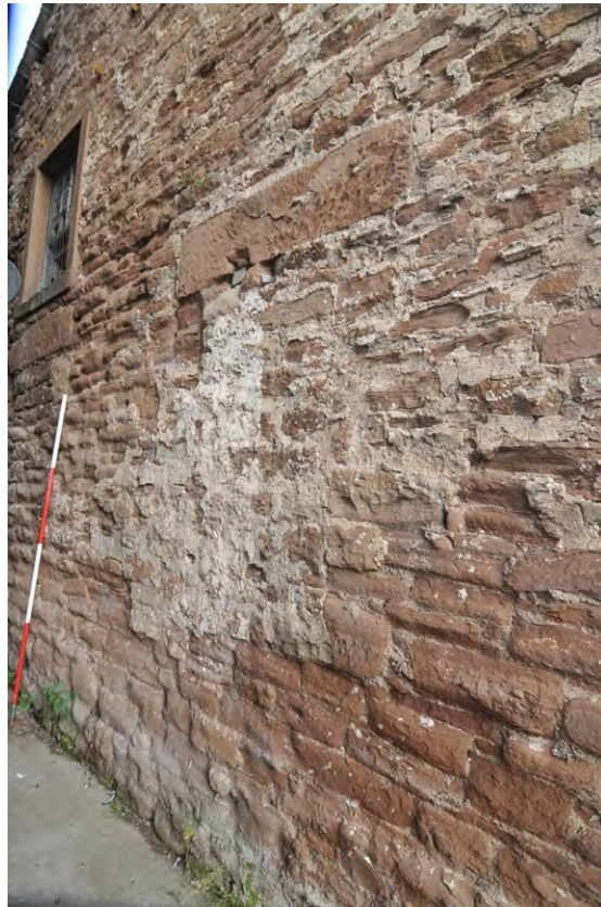
Fig. 19 Exterior south-facing gable wall, blocked windows
