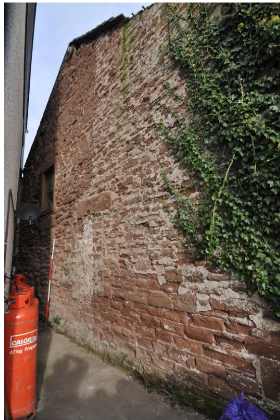
Fig. 18 Exterior south-facing gable wall
