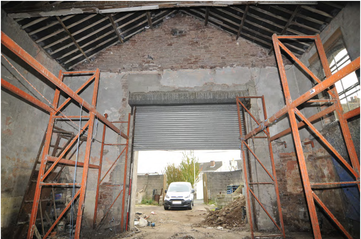
Fig. 5 Room 1, internal south-facing gable wall and roller shutter door
