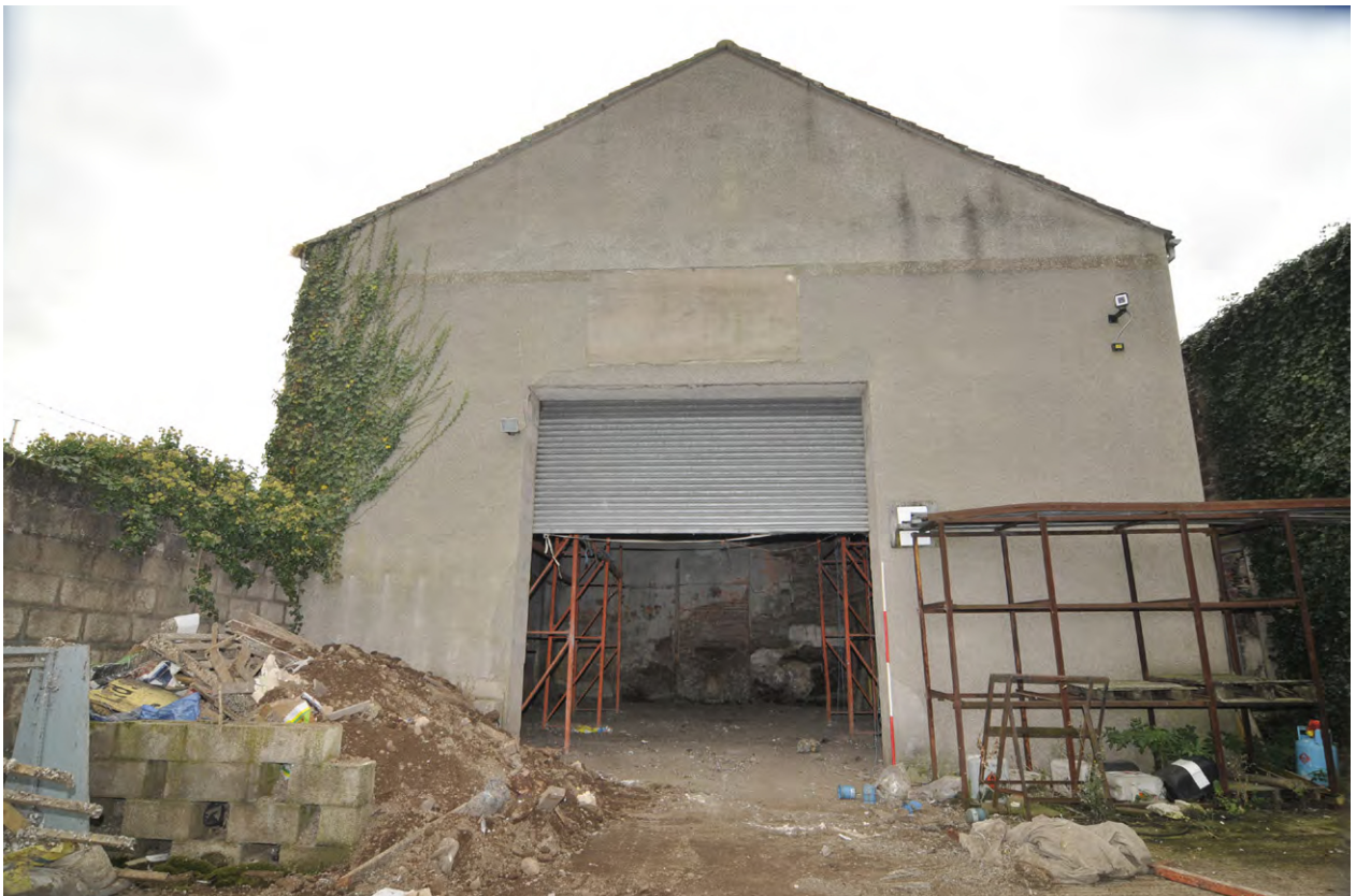
Fig. 16 Exterior north-facing gable wall
