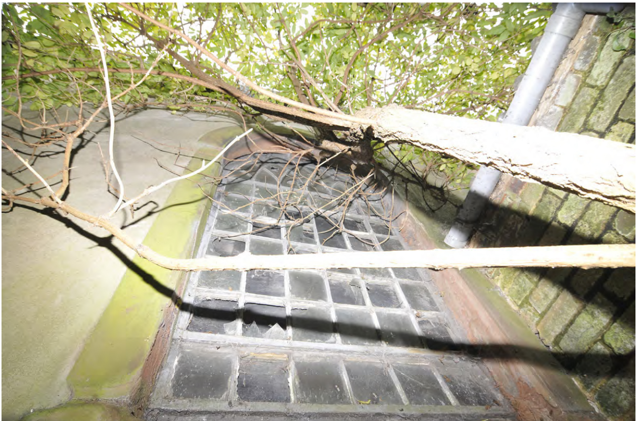
Fig. 20 Exterior west-facing wall with an original 19th century chapel window
