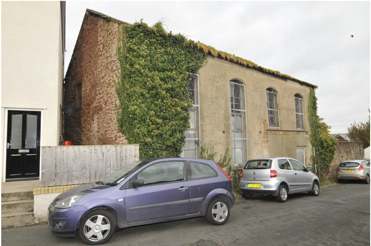
Fig. 17 Exterior east-facing side wall with fenestration
