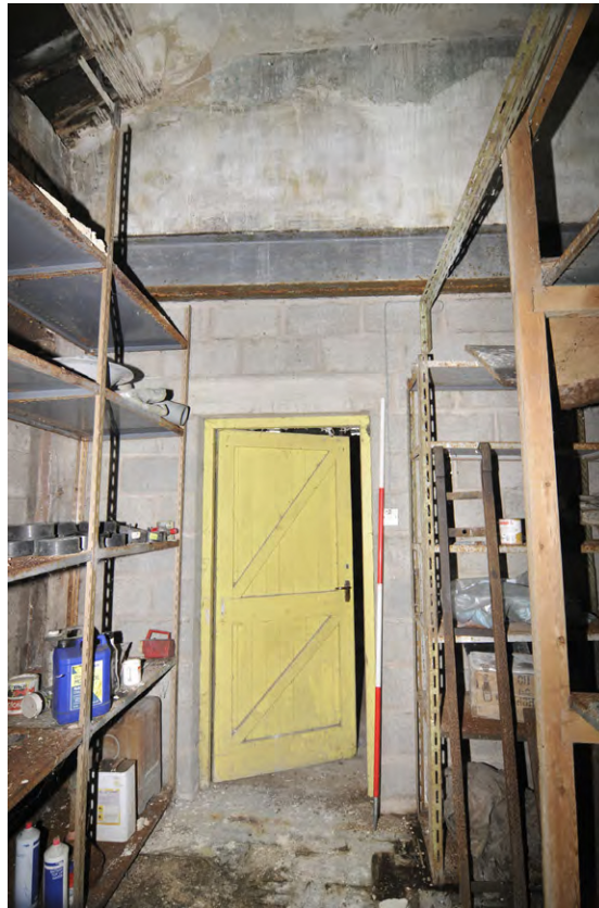
Fig. 13 Room 2, west-facing elevation with inserted plank-built door
