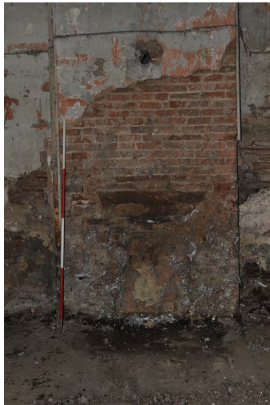
Fig. 8 Room 1, internal north-facing gable, blocked fireplace
