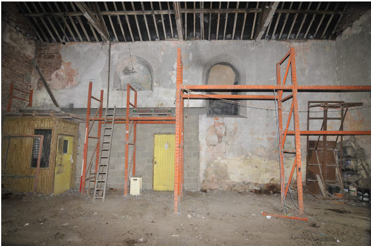
Fig. 10 Room 1, internal east-facing elevation with two blocked round-headed windows
