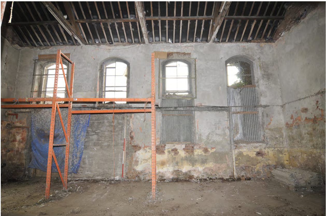
Fig. 6 Room 1, internal west-facing elevation (side wall) with round-headed windows
