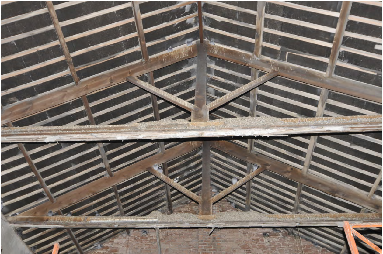
Fig. 11 Room 1, king-post roof trusses
