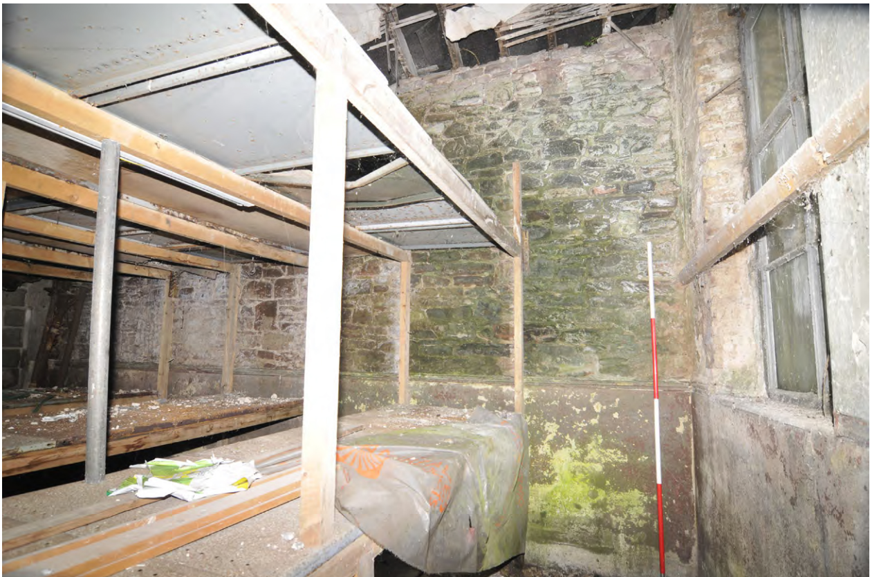
Fig. 14 Room 2, north-facing elevation, rubble-built wall
