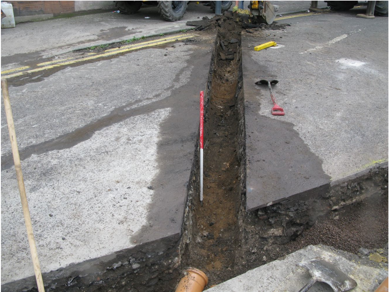
Fig. 4 - Gully trench showing possible natural sand at base
