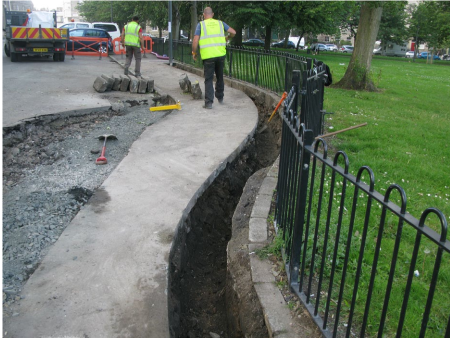
Fig. 2 - General shot of duct trench
