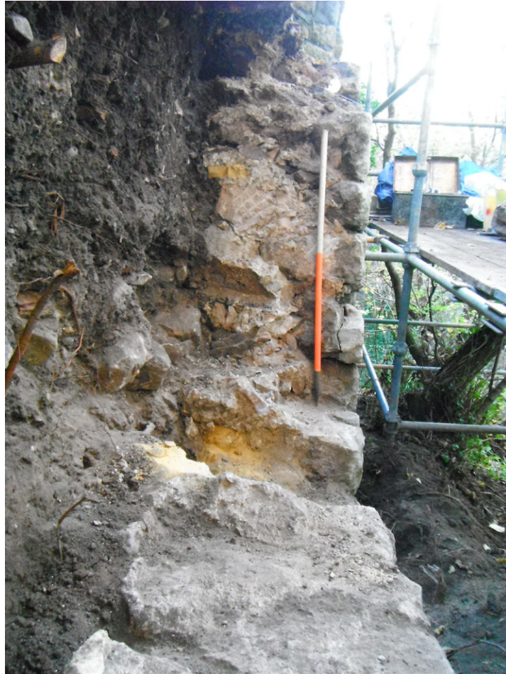
Fig. 6 - North facing section through the retaining wall (005)
