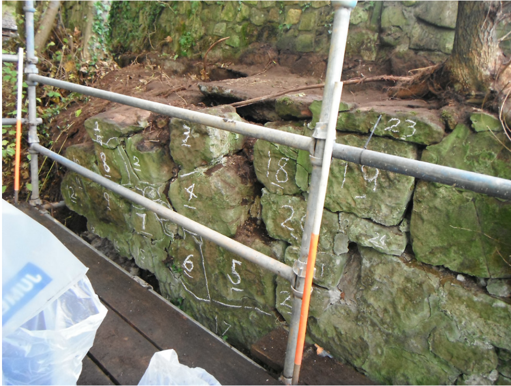
Fig. 4 - Numbering of the stones in the detached portion (006) of the retaining wall
