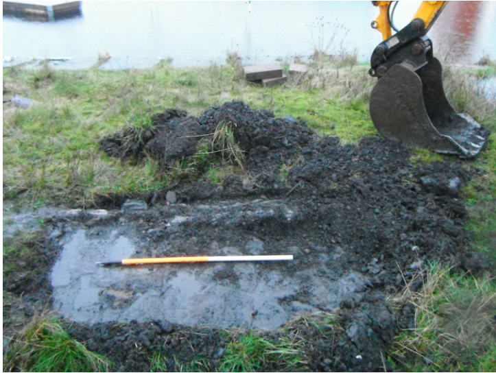
Fig. 5 - TP2 from south
