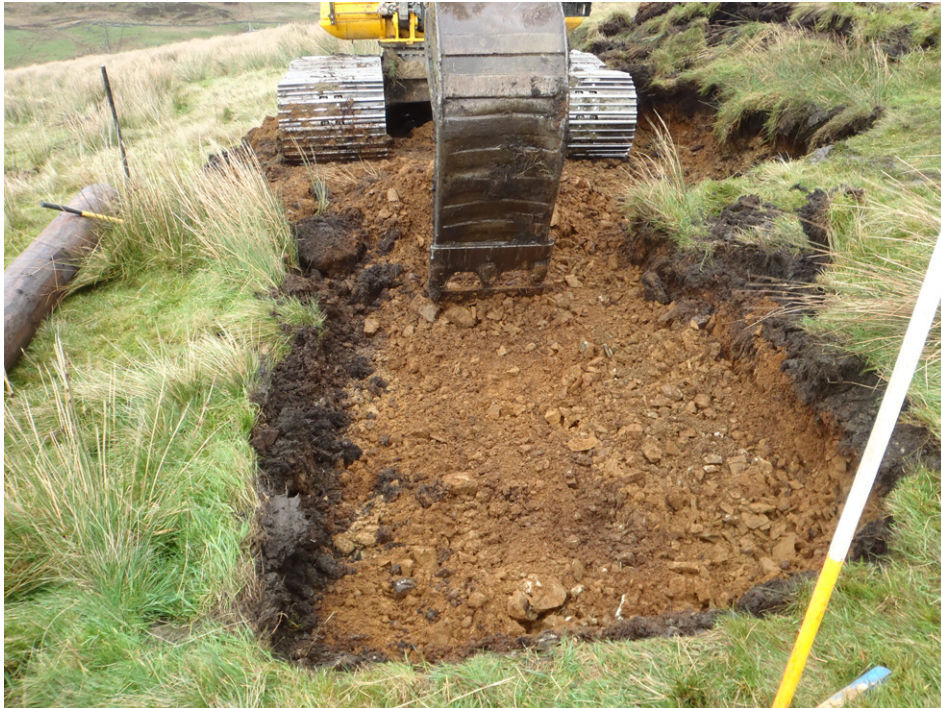
Fig. 12 - Foundation for pole 107
