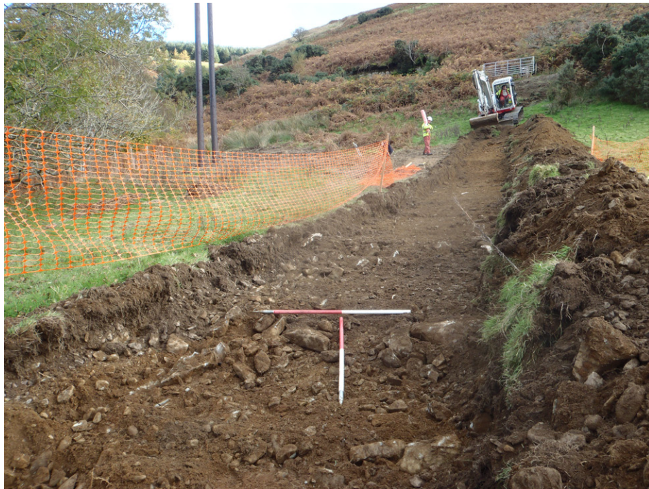
Fig. 11 - Area showing pole no. 1 and stripped area designated for cabling
