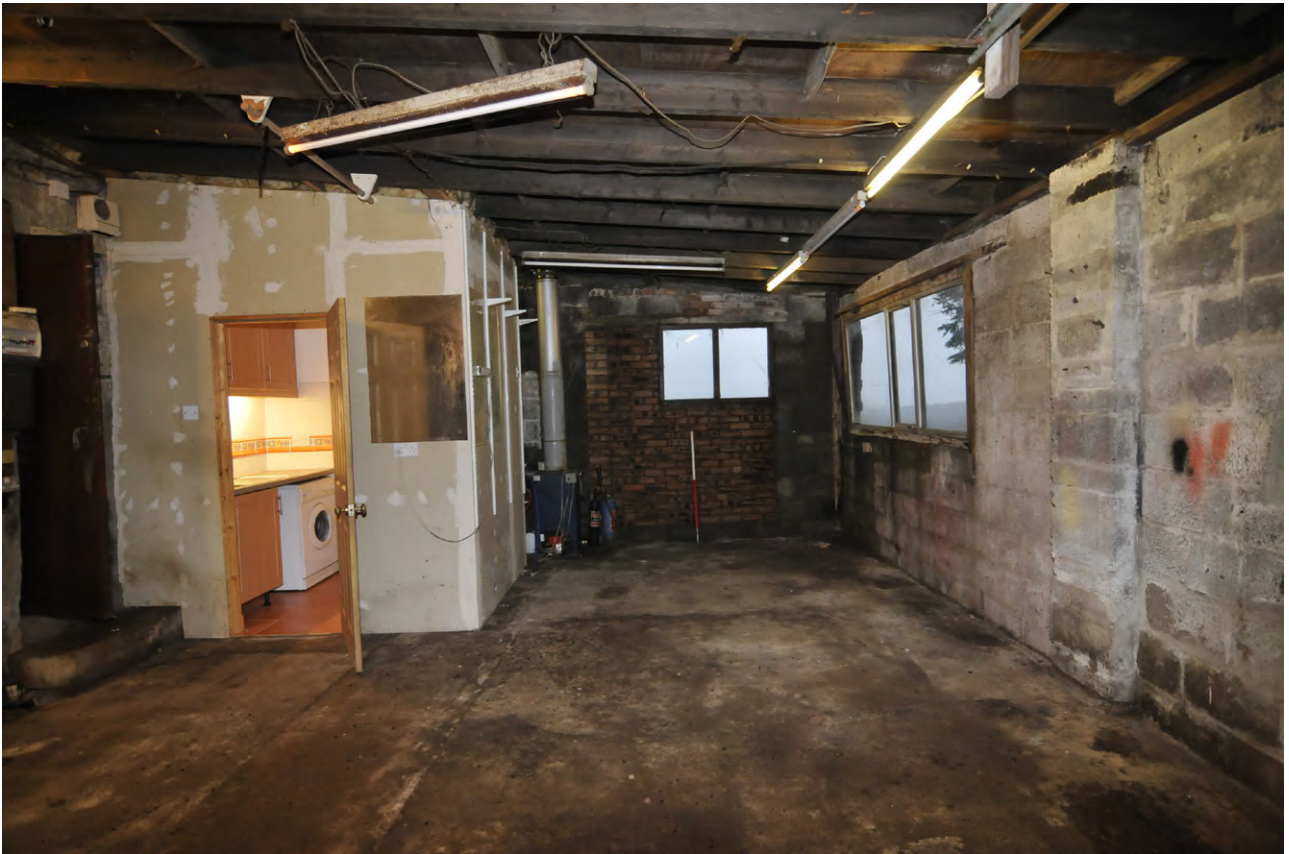
Fig. 7 Room 1 Garage, interior view (030)
