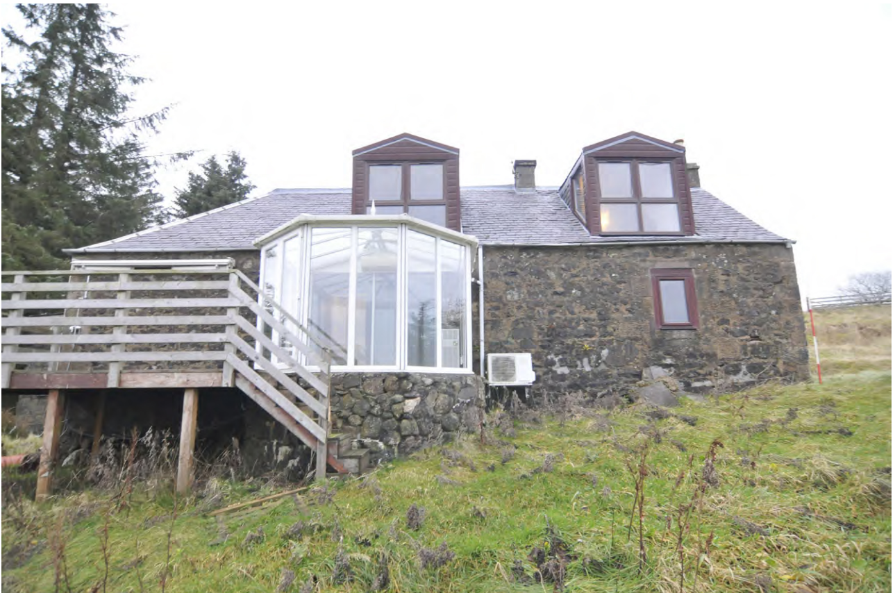
Fig. 6 West-facing elevation of the cottage (007)
