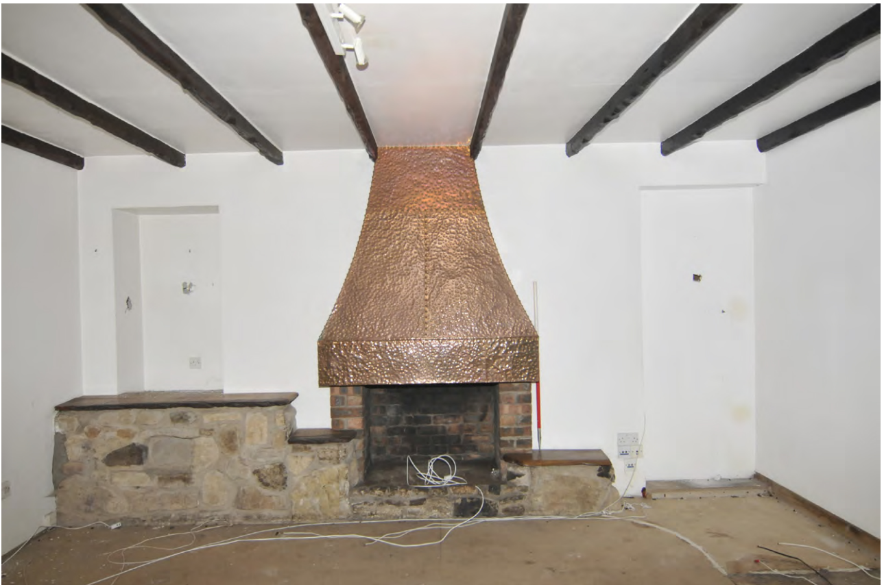
Fig. 10 Room 7 Living Room fire place (022)
