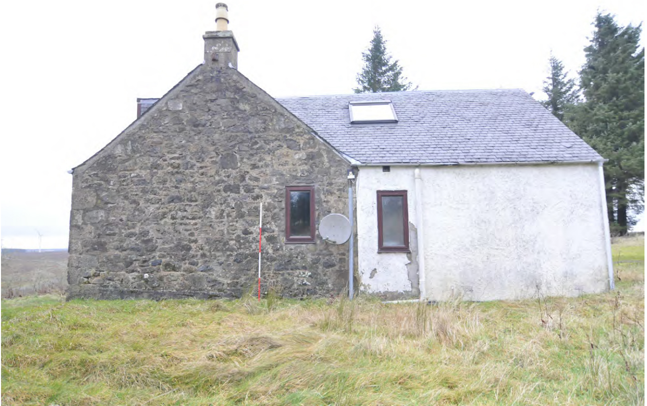
Fig. 5 South-facing elevation of the cottage (005)
