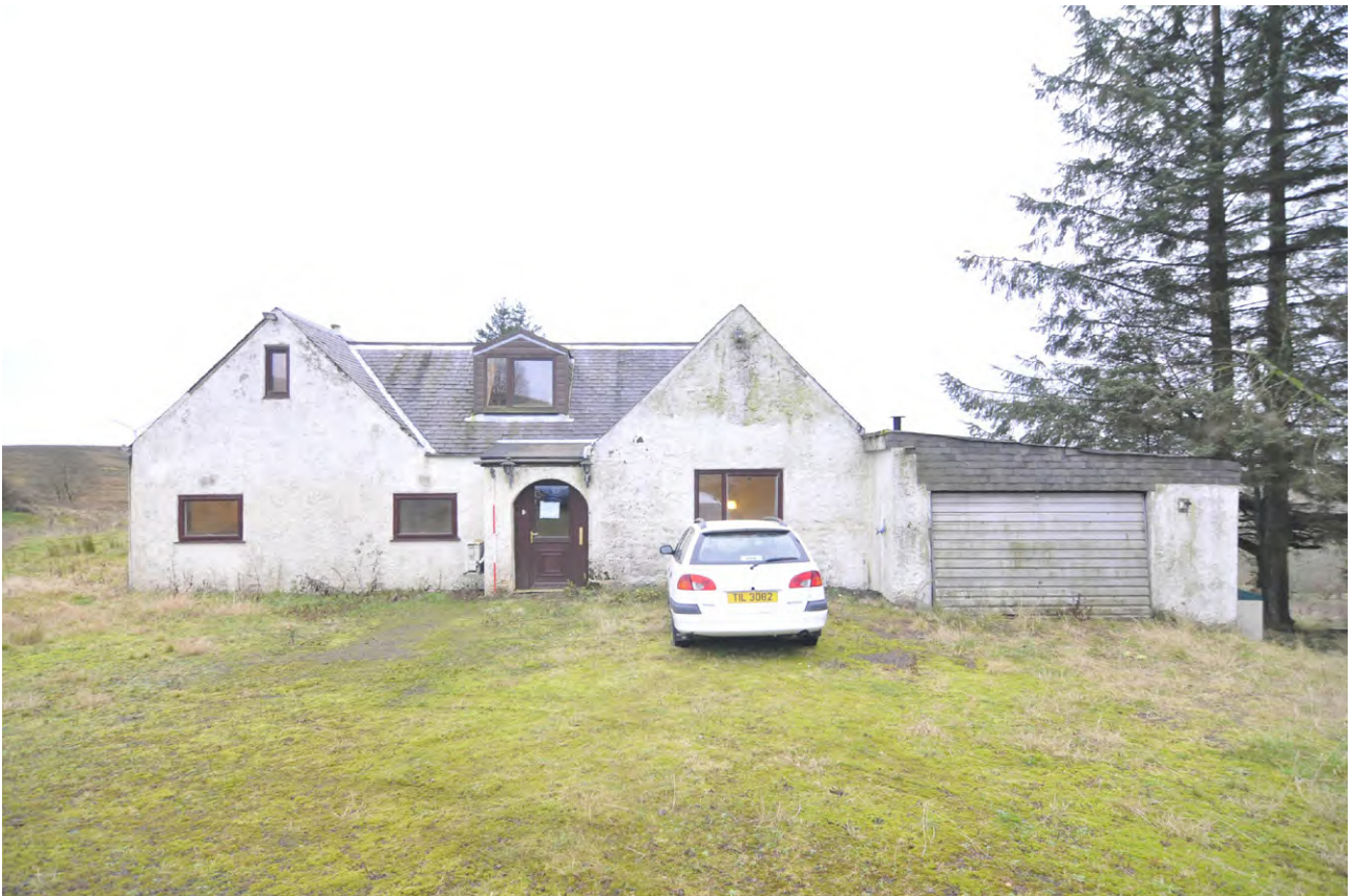
Fig. 4 East-facing elevation of the cottage (001)
