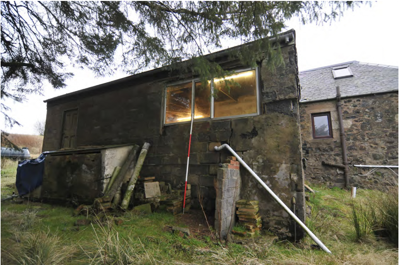
Fig. 3 North-facing elevation of the cottage and garage (012)
