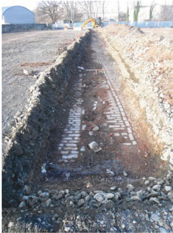
Fig. 35 - General view of Trench 6 from the south-east
