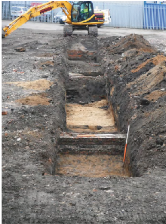
Fig. 23 - Wall 301 from the south-east. Same as wall 101 in Trench 1
