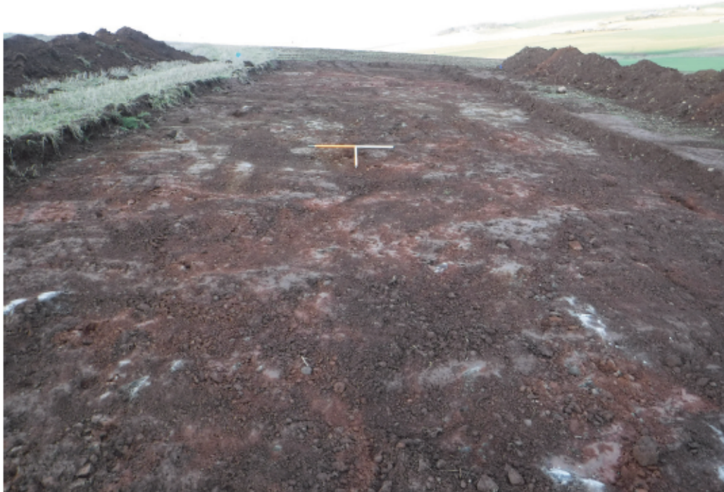
Fig. 2 - General post-excavation shot of haul road
