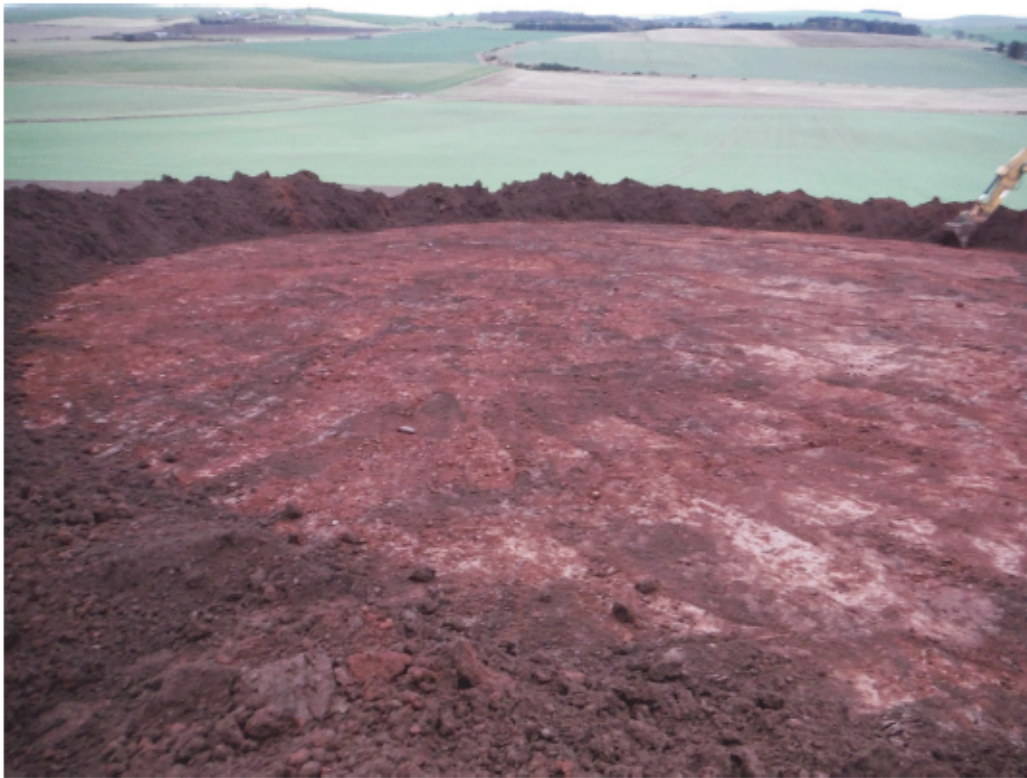
Fig. 8 - General post-excitation shot of Turbine 1 base
