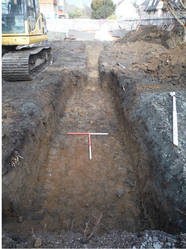
Fig. 6 - Wider foundation trench for bay window from south
