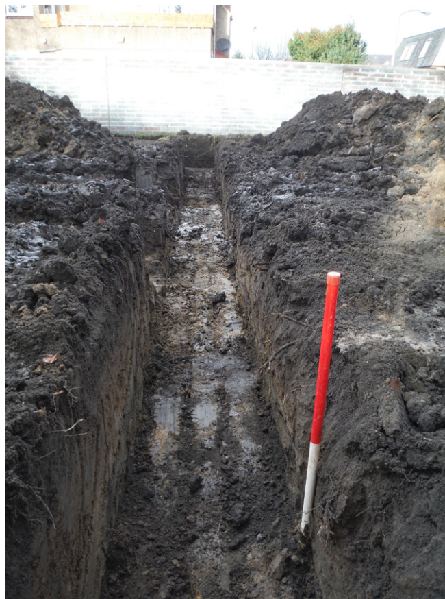
Fig. 3 - Example of foundation trench from south
