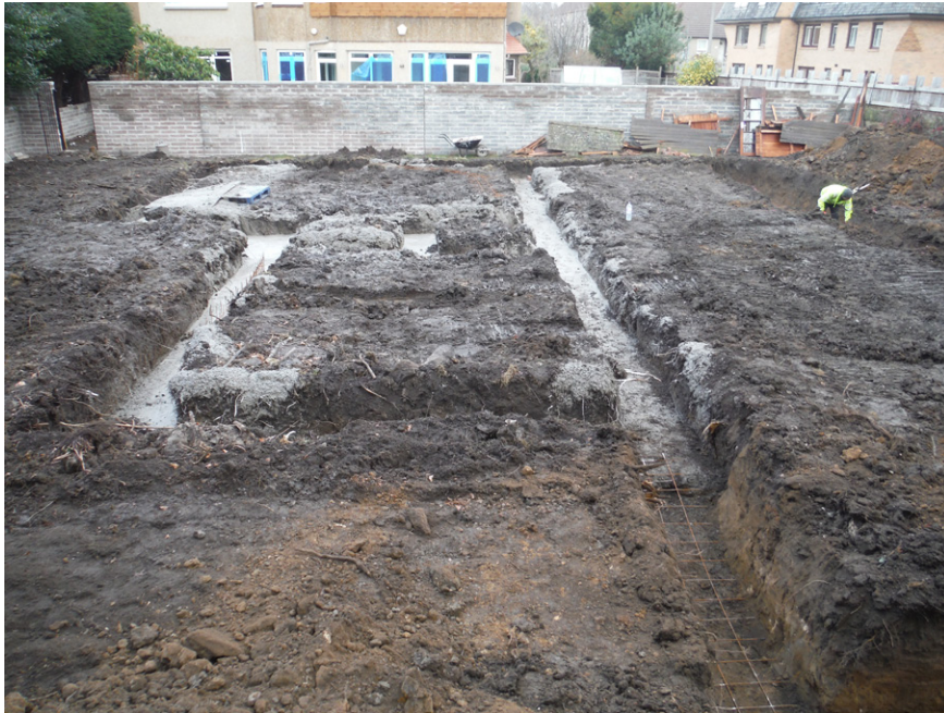
Fig. 4 - General site shot from south
