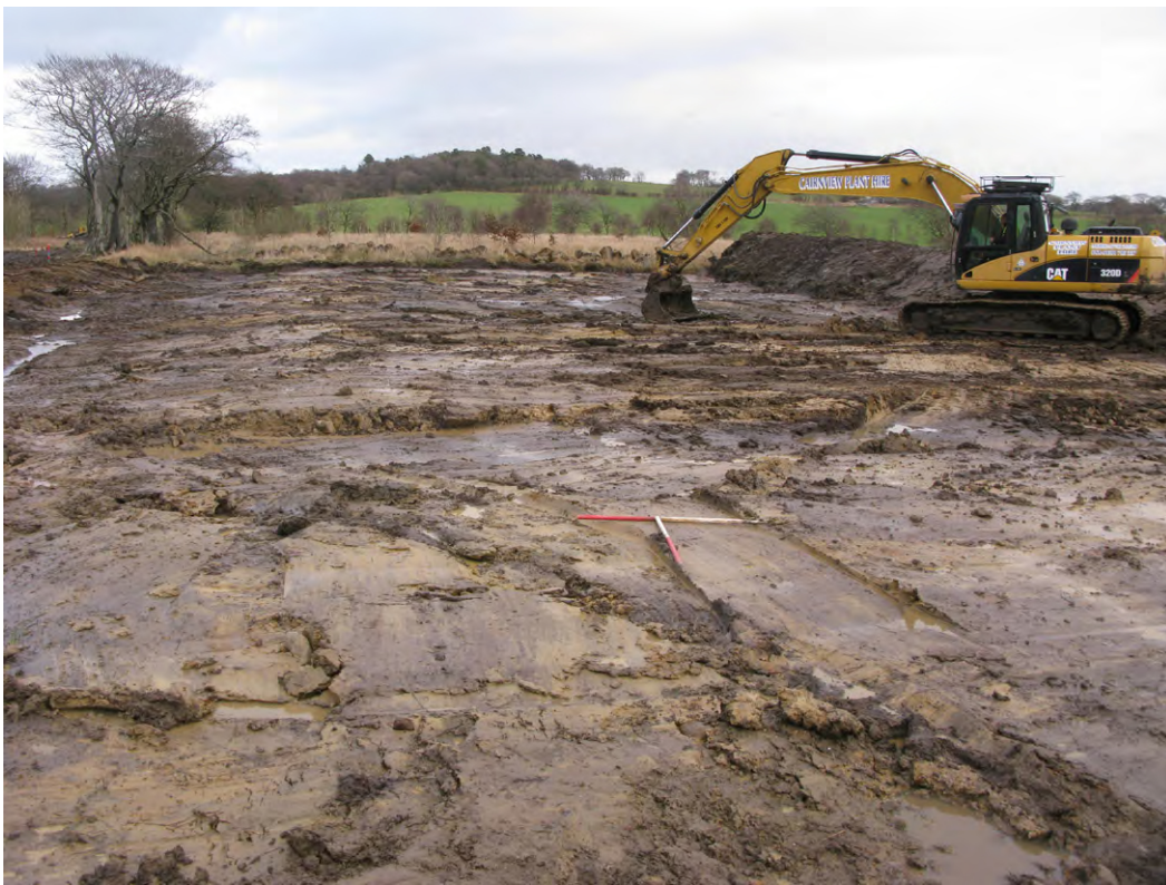
Fig. 2 General Post ex of Turbine 2 crane pad looking NE
