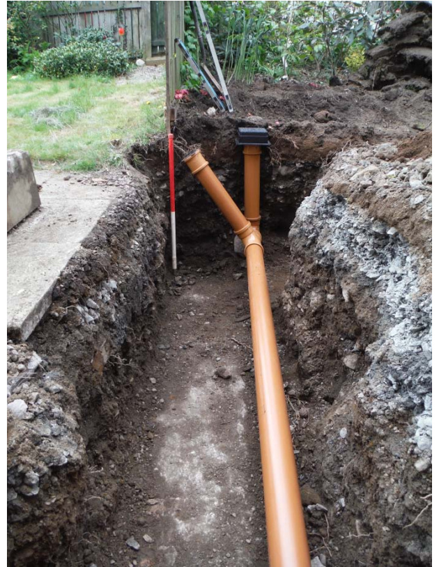
Fig. 3 - Southernmost foundation trench excavated to concrete 003
