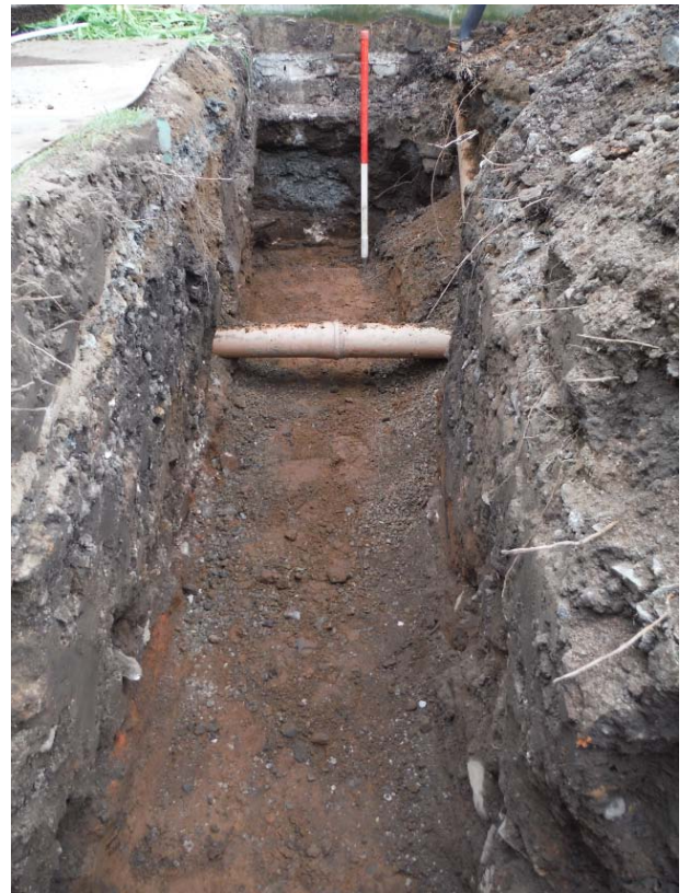
Fig. 5 - Northernmost foundation trench excavated to natural substratum
