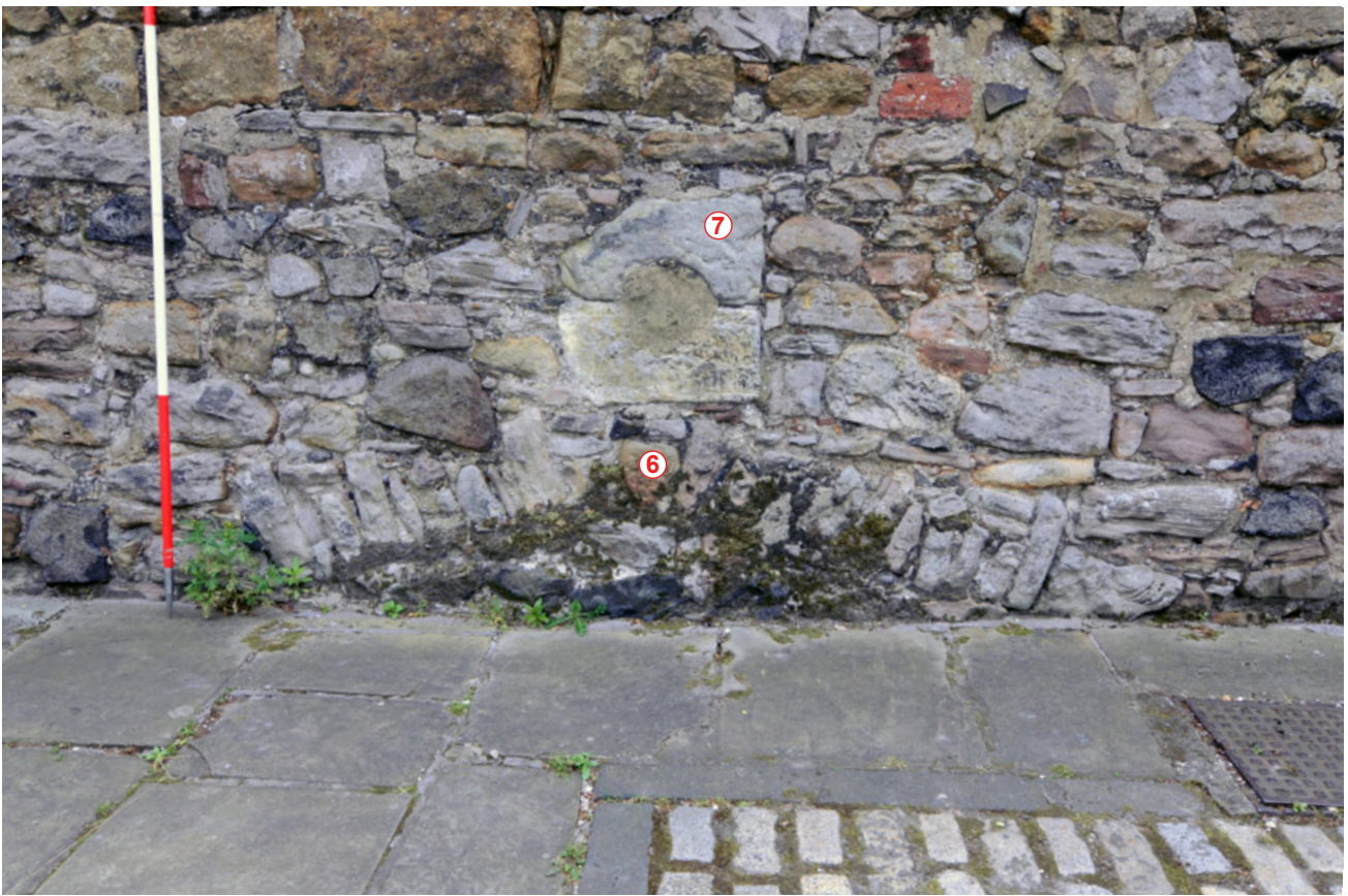
Fig. 10 - North-facing elevation, blocked segmented arch (Feature 6) and gun loop? above (Feature 7).
