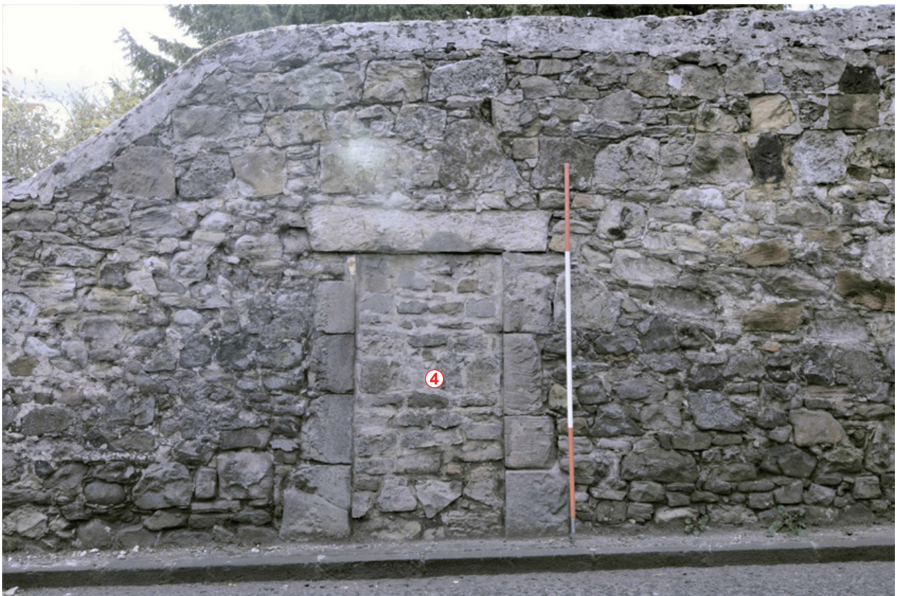
Fig. 8 - North-facing elevation, blocked doorway (Feature 4).
