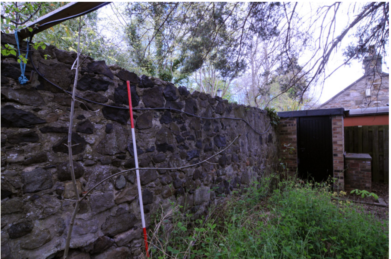
Fig. 16 - South-facing elevation, general view of the wall terminus.
