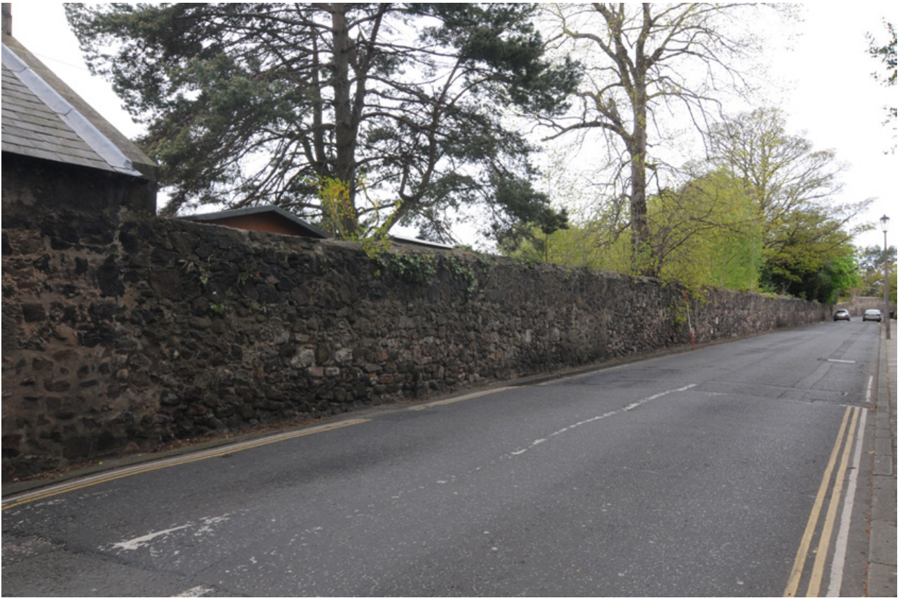
Fig. 4 - North-facing elevation, east end, general view.
