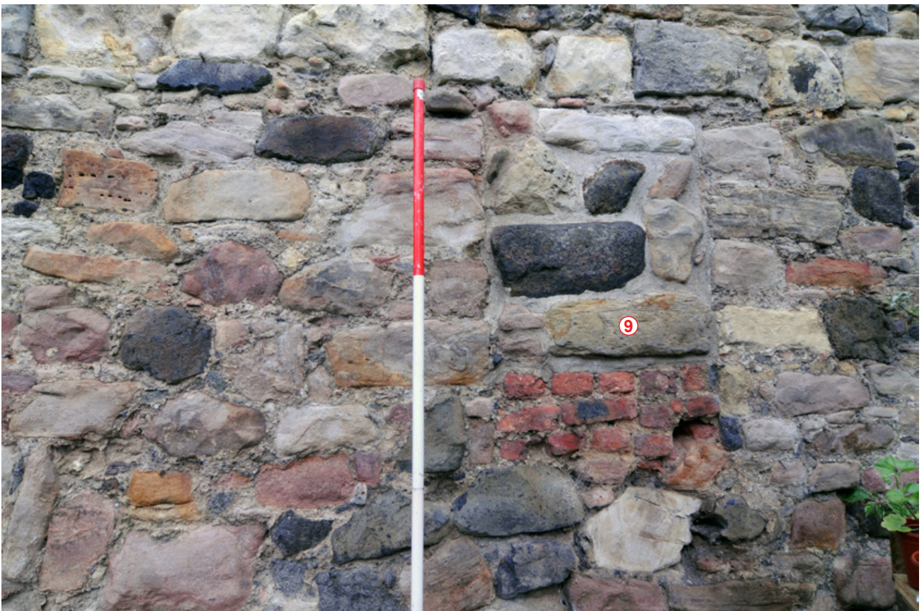
Fig. 13 - South-facing elevation, blocked bee hole (Feature 9).
