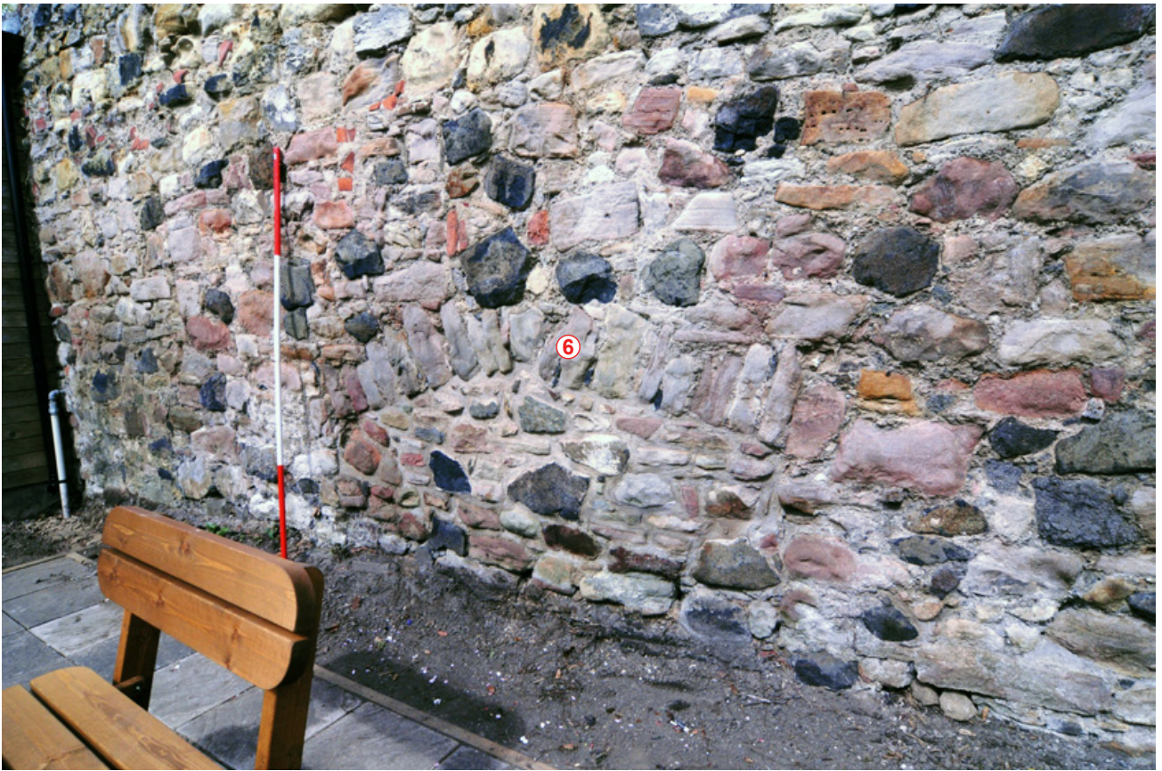
Fig. 12 - South-facing elevation, segmented arch (Feature 6).
