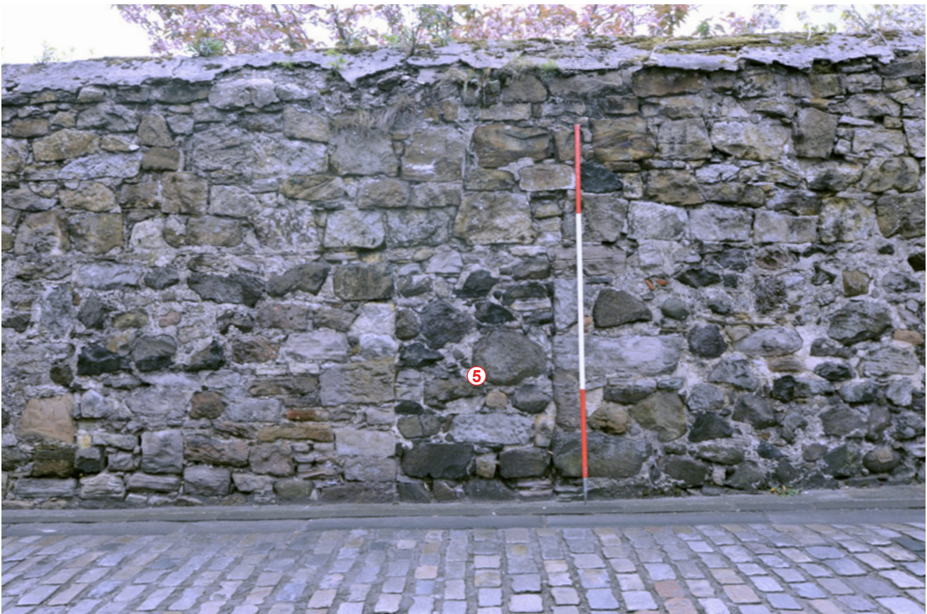
Fig. 9 - North-facing elevation, blocked opening (Feature 5).
