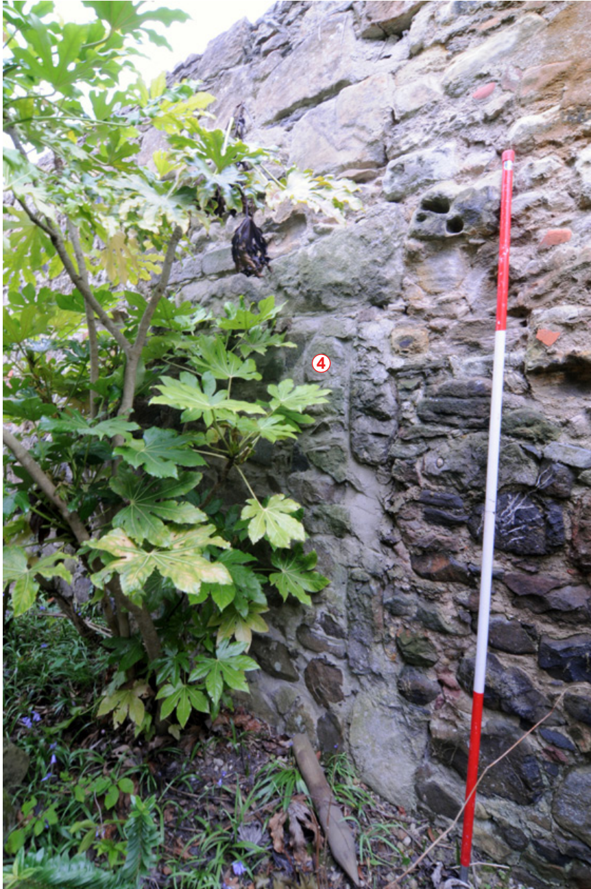
Fig. 14 - South-facing elevation, blocked door Feature 4).
