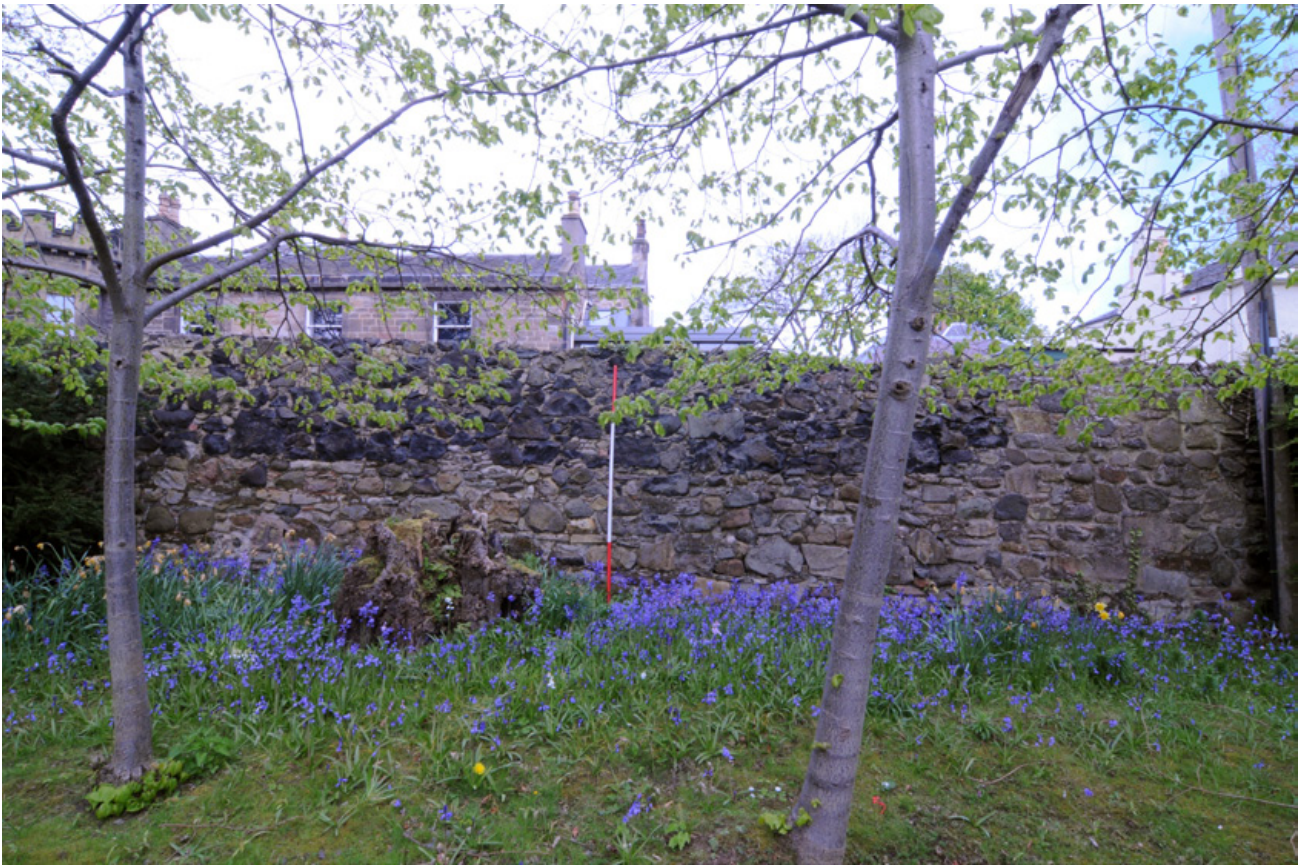
Fig. 15 - South-facing, random rubble and whinstone at Section A-B.
