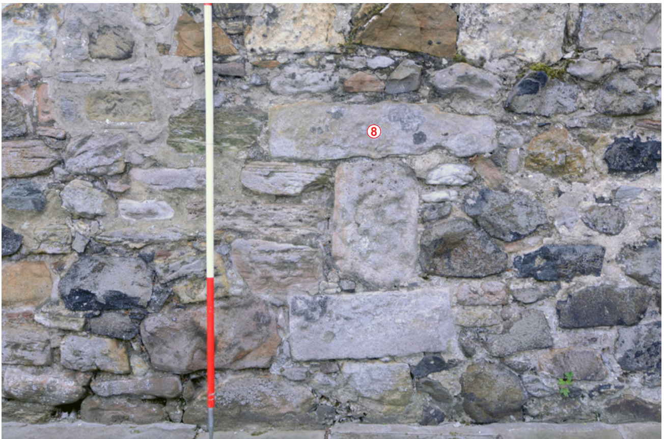
Fig. 11 - North-facing elevation, irregular stonework (Feature 8).
