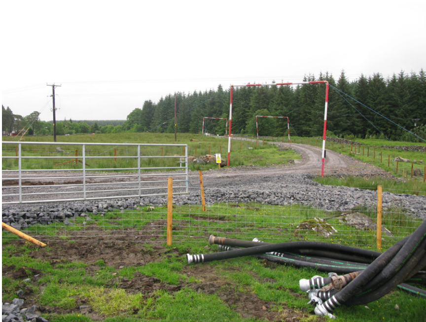
Fig. 3 - Floated access track
