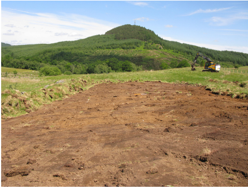
Fig. 2 - Initial topsoil strip exposing natural deposits
