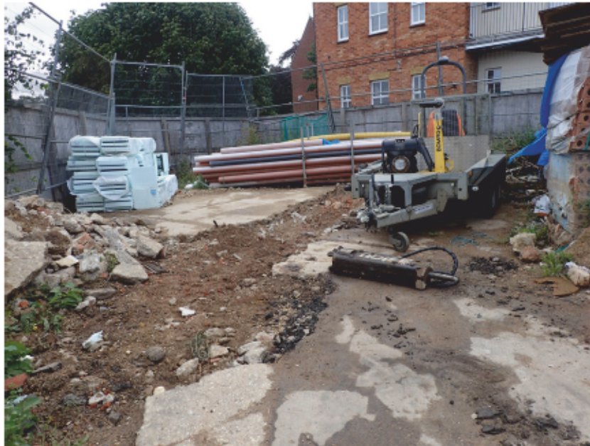
Fig. 2 - Site prior to commencement of works, taken from W
