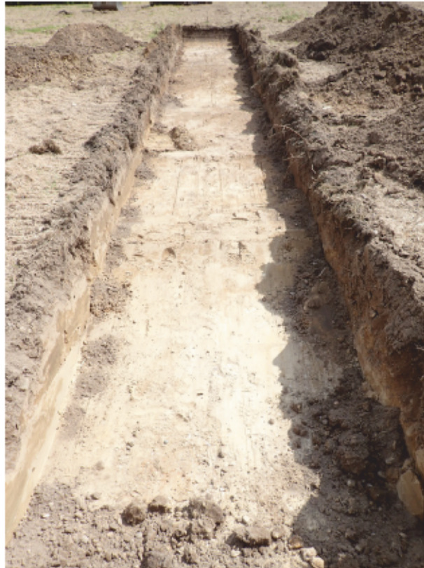
Fig. 6 - Trench 5, taken from NW
