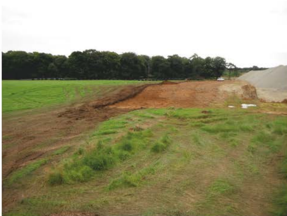
Fig. 14 - General view of the site from the SW
