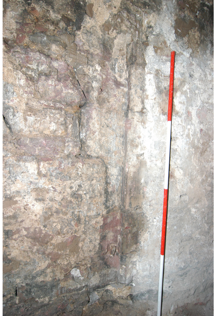
Fig. 11 - The remains of a blocked doorway in Room G06, with an iron door hanger
