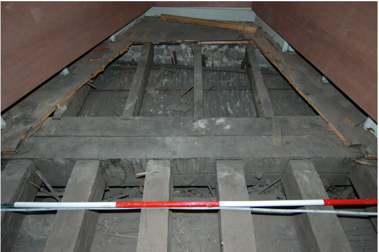
Fig. 26 - Detailed shot of the load-bearing fitch-beam in Room F10
