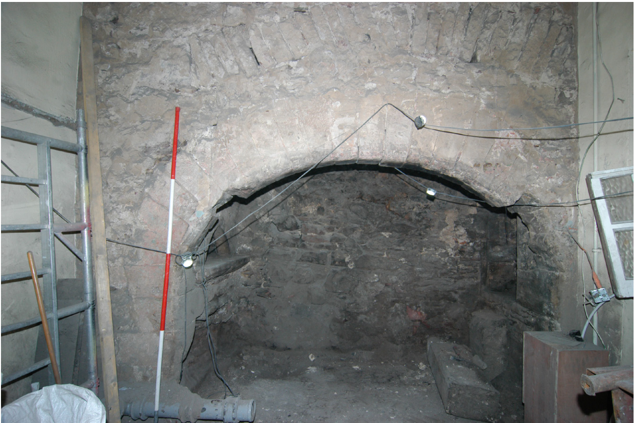
Fig. 16 - The kitchen fireplace after the removal of its later insertions
