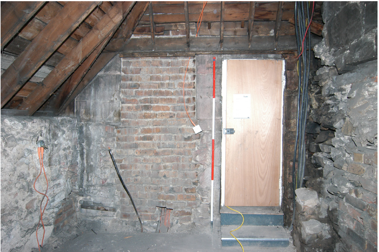
Fig. 24 - A late 16th century blocked doorway in Room F04, south-facing elevation
