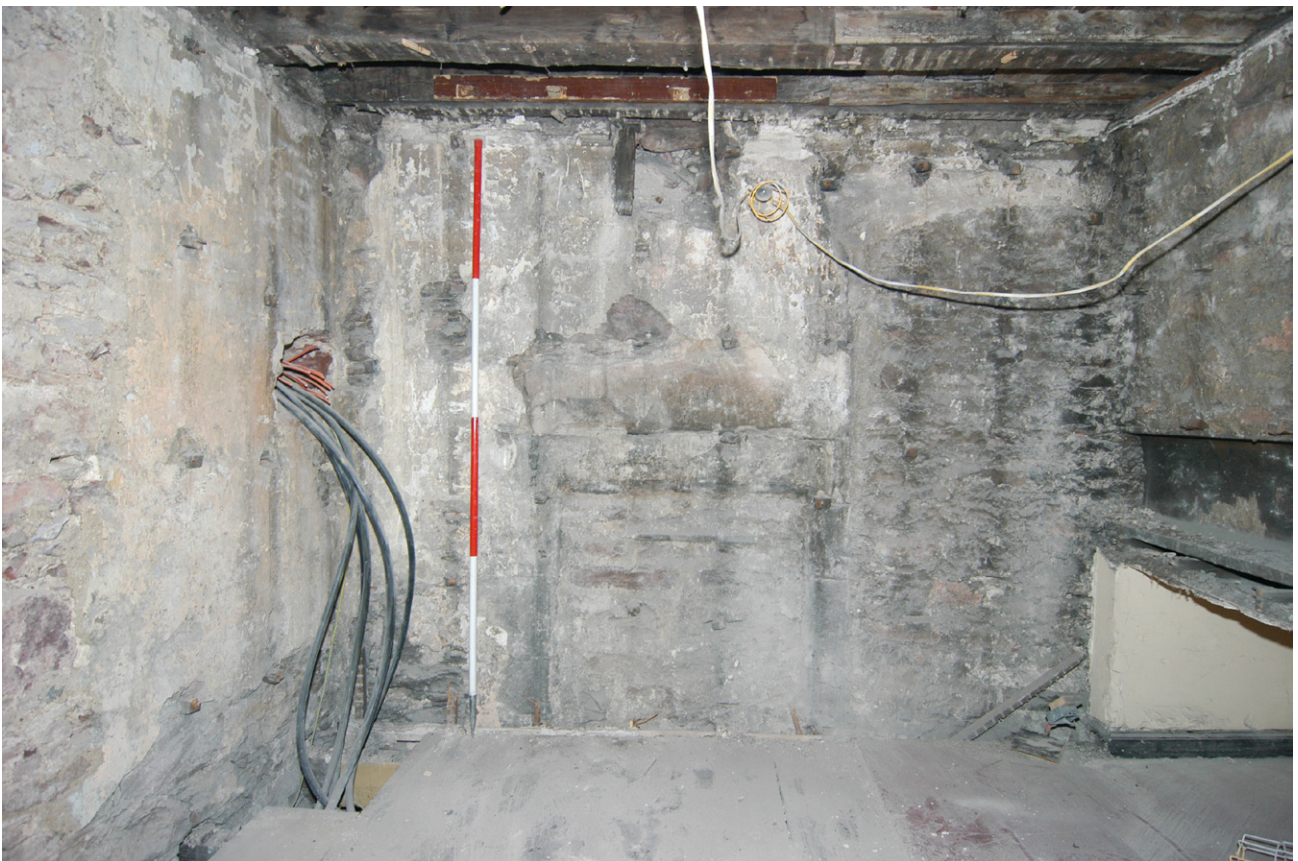
Fig. 27 - The blocked fireplace and press in Room F12, west-facing elevation
