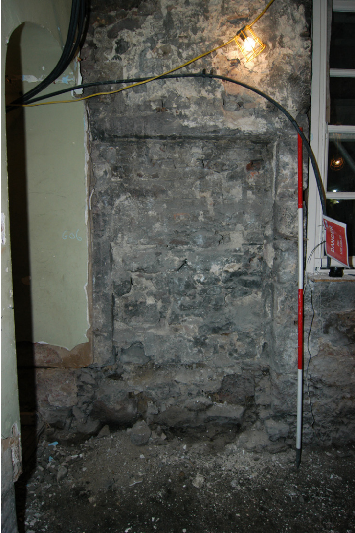
Fig. 10 - A blocked doorway in Room G06 on the east-facing elevation
