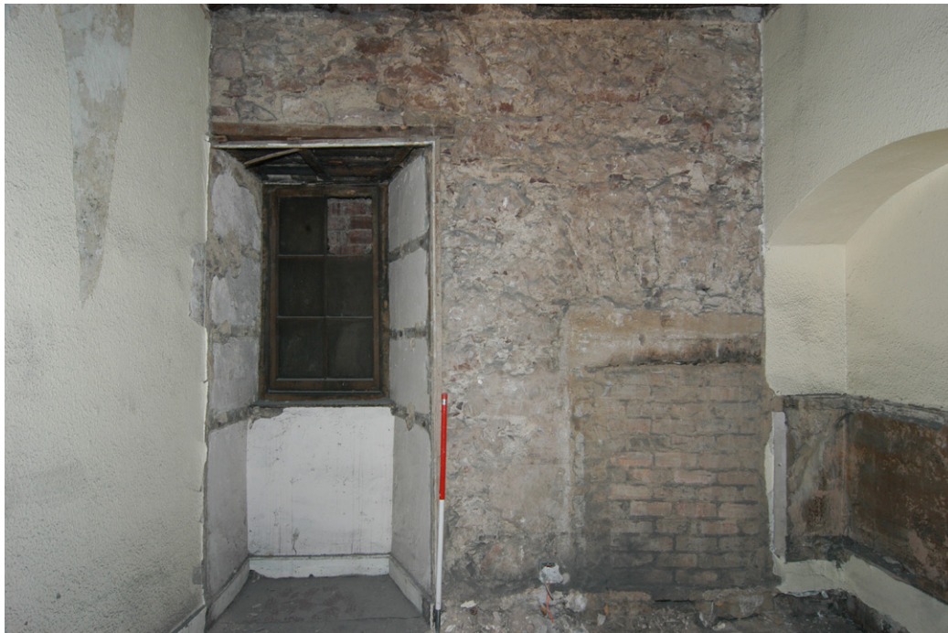
Fig. 33 - Exposed blocked window and fireplace in Room S08
