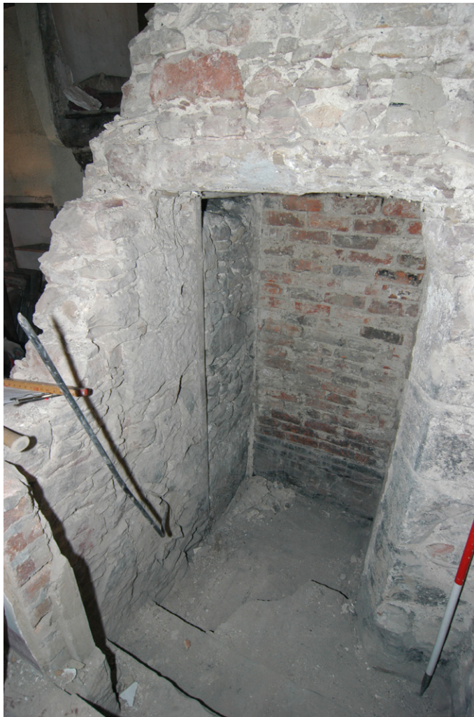
Fig. 32 - An early rubble-blocked doorway in Room S07 with chamfer moulding door surrounds
