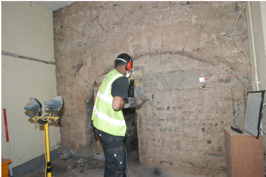
Fig. 15 - Breaking out the blocking work within the inserted 19th century fireplace
