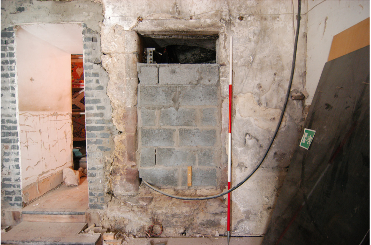
Fig. 4 - An early 16th century doorway in Basement Room B02 with modern blocking
