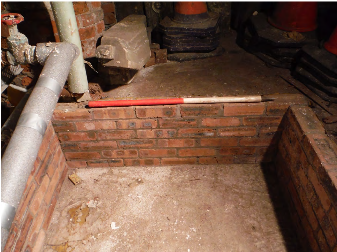
Fig. 8 - Existing brick-lined pit (pre-excavation)
