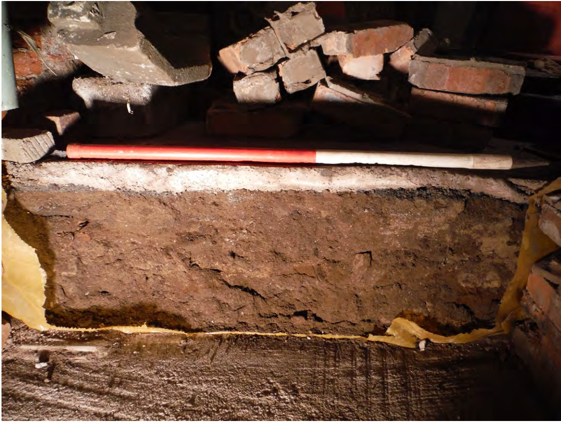
Fig. 9 - Existing brick-lined pit (WSW-facing section)
