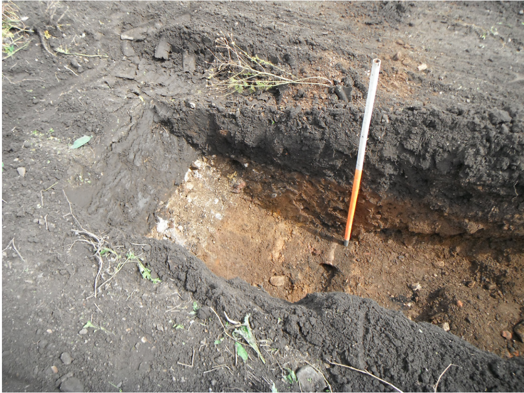
Fig. 4 Test-pit 324 with possible wall foundation trench
