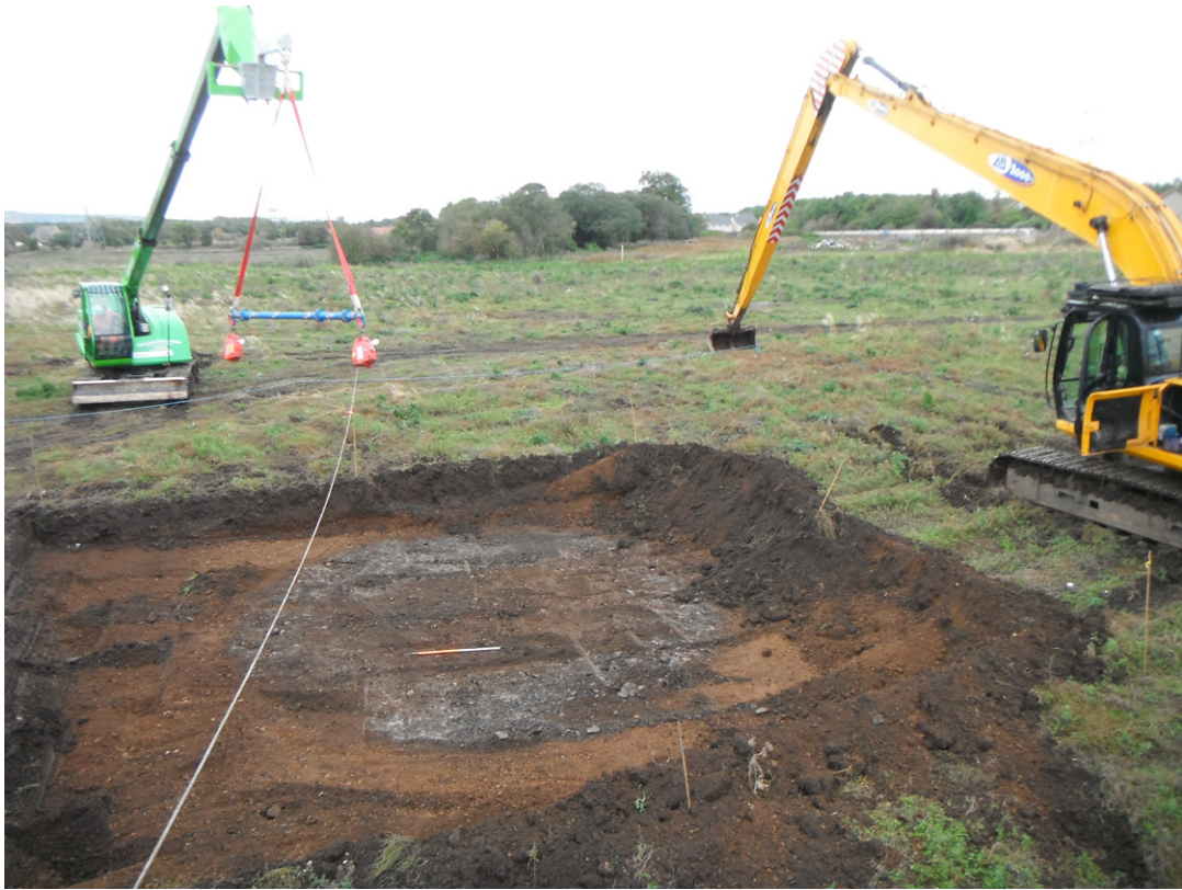
Fig. 8 Shaft Investigation Trench SH509 showing circular feature 032
