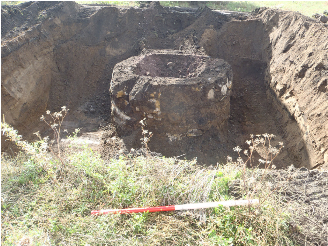
Fig. 6 Shaft Investigation Trench SH515 showing stone capping 021
