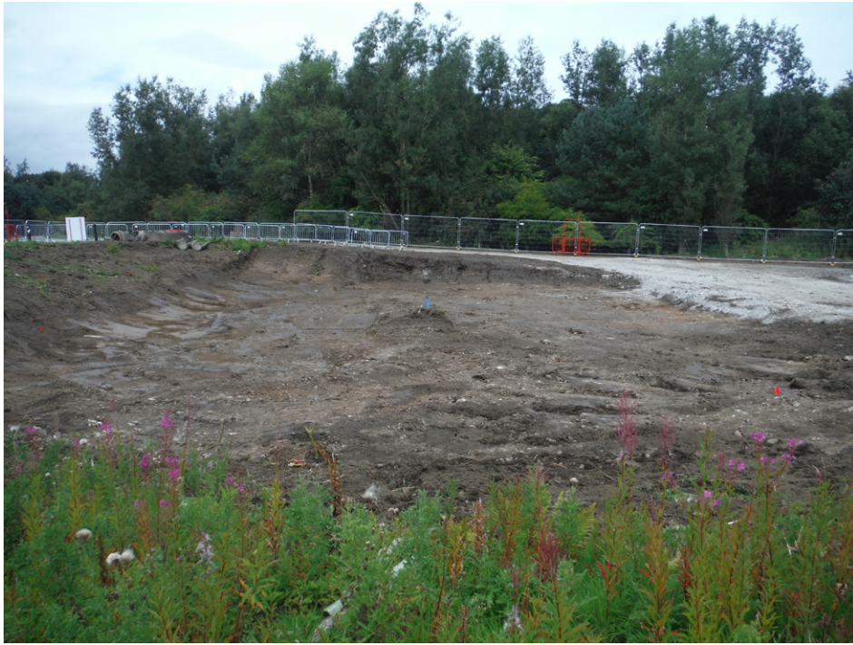
Fig. 6 - The Storage Area stripped from the East
