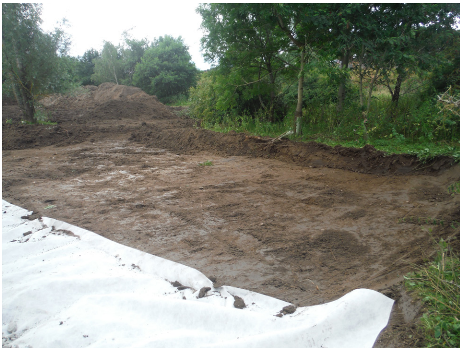
Fig. 3 - The Parking Area stripped to foundation level from the South-East
