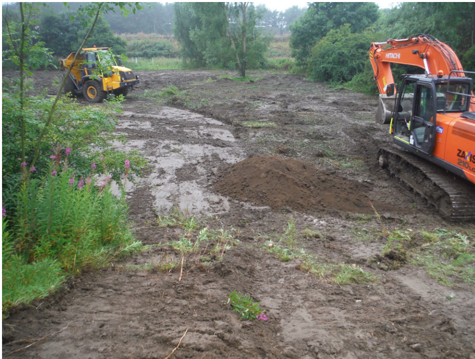
Fig. 2 - The Parking Area after vegetation clearance
