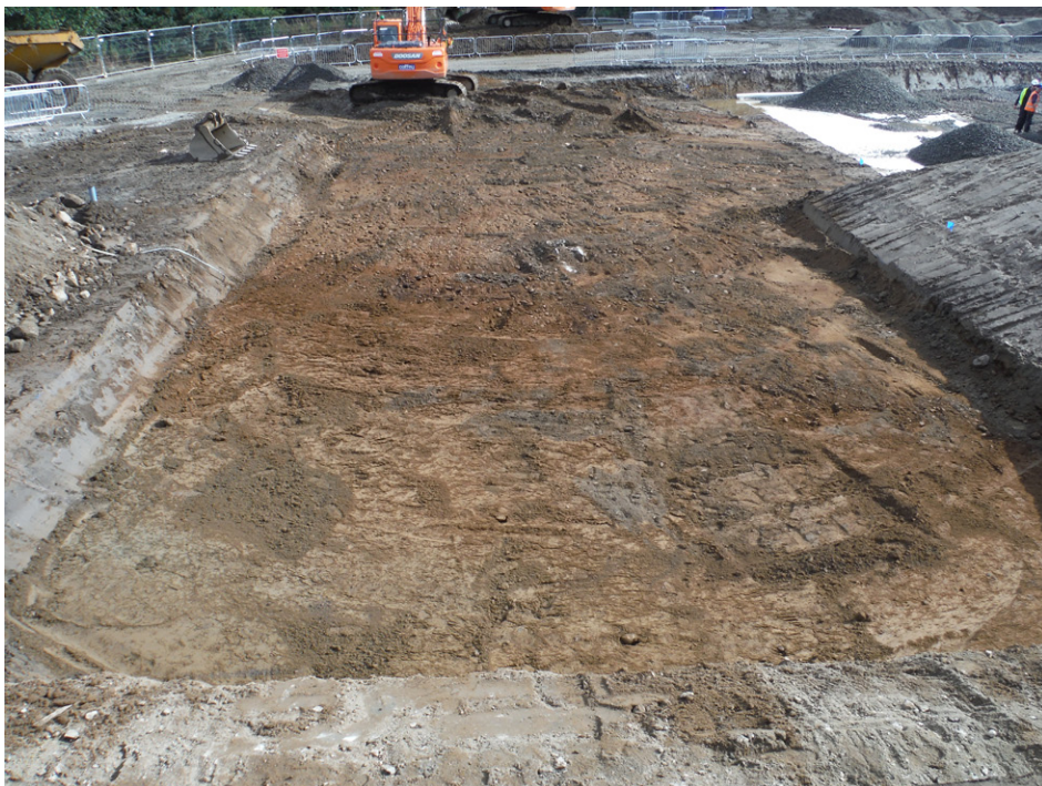
Fig. 5 - The northern end of the NEREDA Tank area from the West
