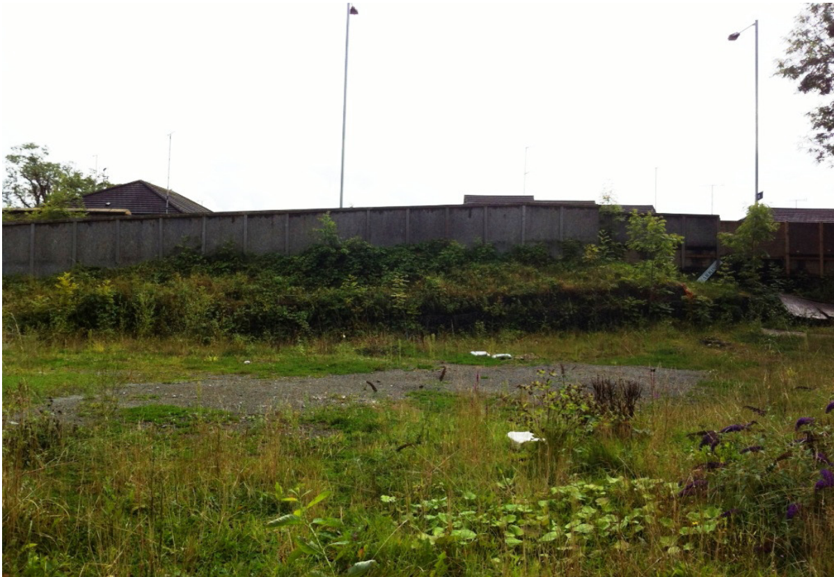
Plate 2: Gabion Wall and Revetment towards School Brow, looking south
