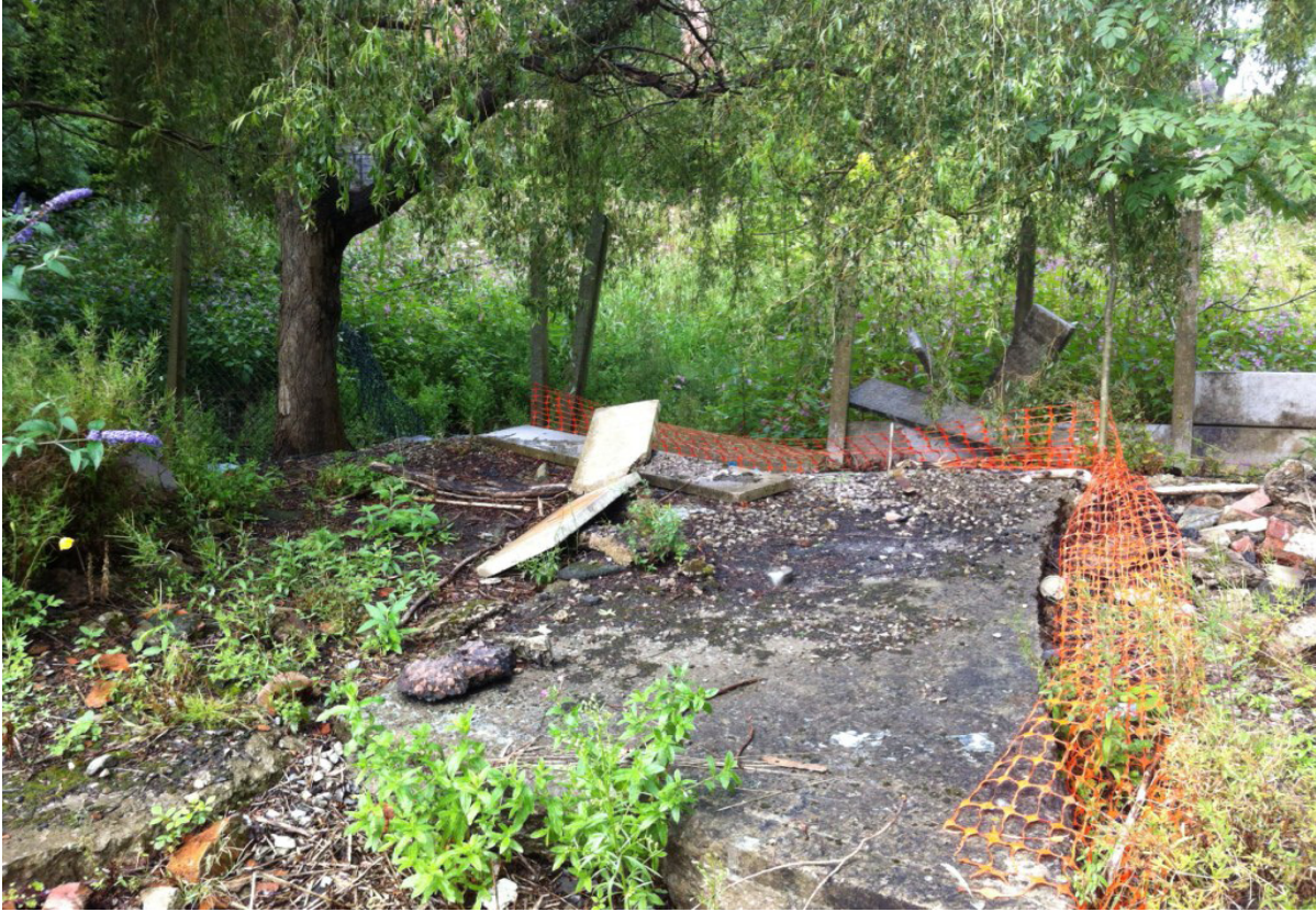
Plate 1: Concrete house platform, looking north
