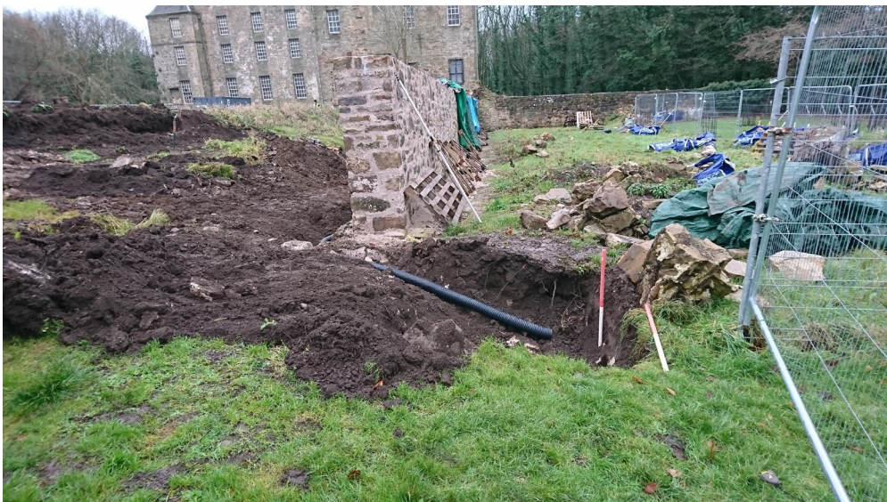
Fig. 4 - Post-excitation view of watching brief area
