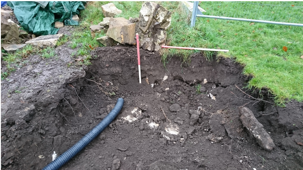
Fig. 3 - Excavated area for sump and drainage pipe
