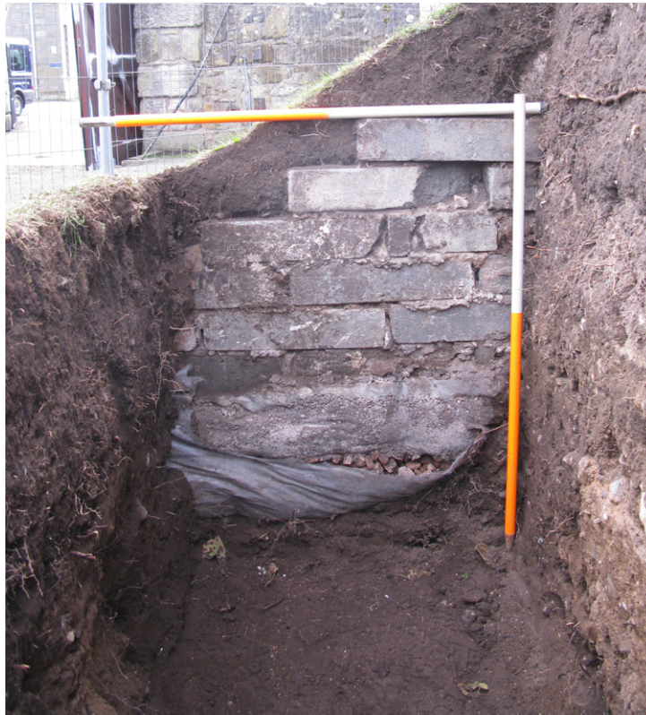
Fig. 5 - Breeze block shoring in TP1
