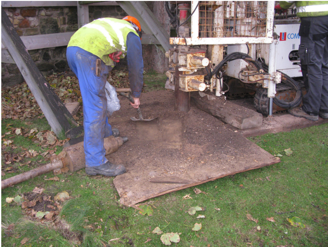
Fig. 9 - Drilling activities showing extraction of soil
