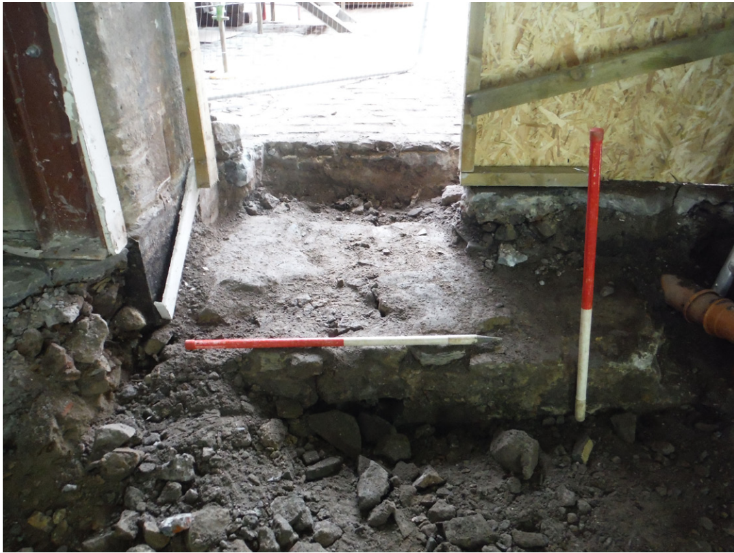
Fig. 7 - Foundation 003 for existing building
