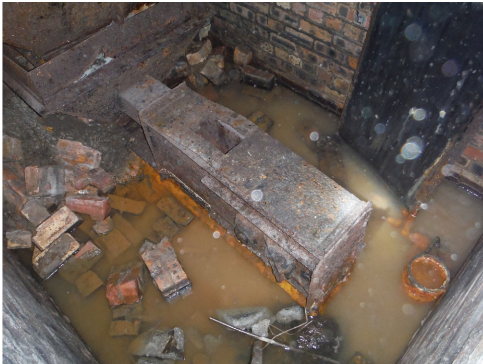
Fig. 4 - Hopper and associated machinery within brick-built pit 013
