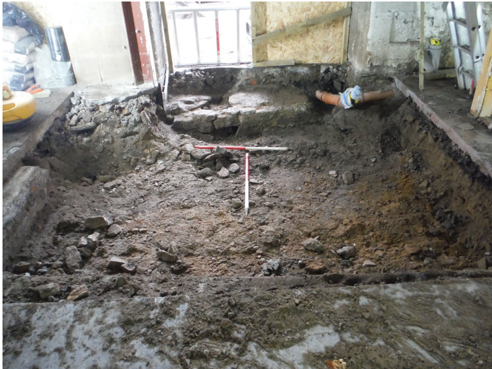
Fig. 6 - General shot of Trench 2
