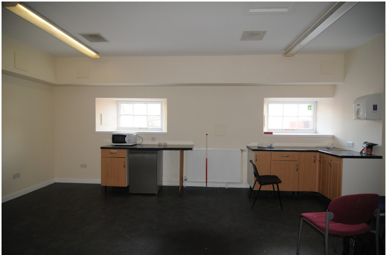
Fig. 14 - Unit 10 First floor mess room
