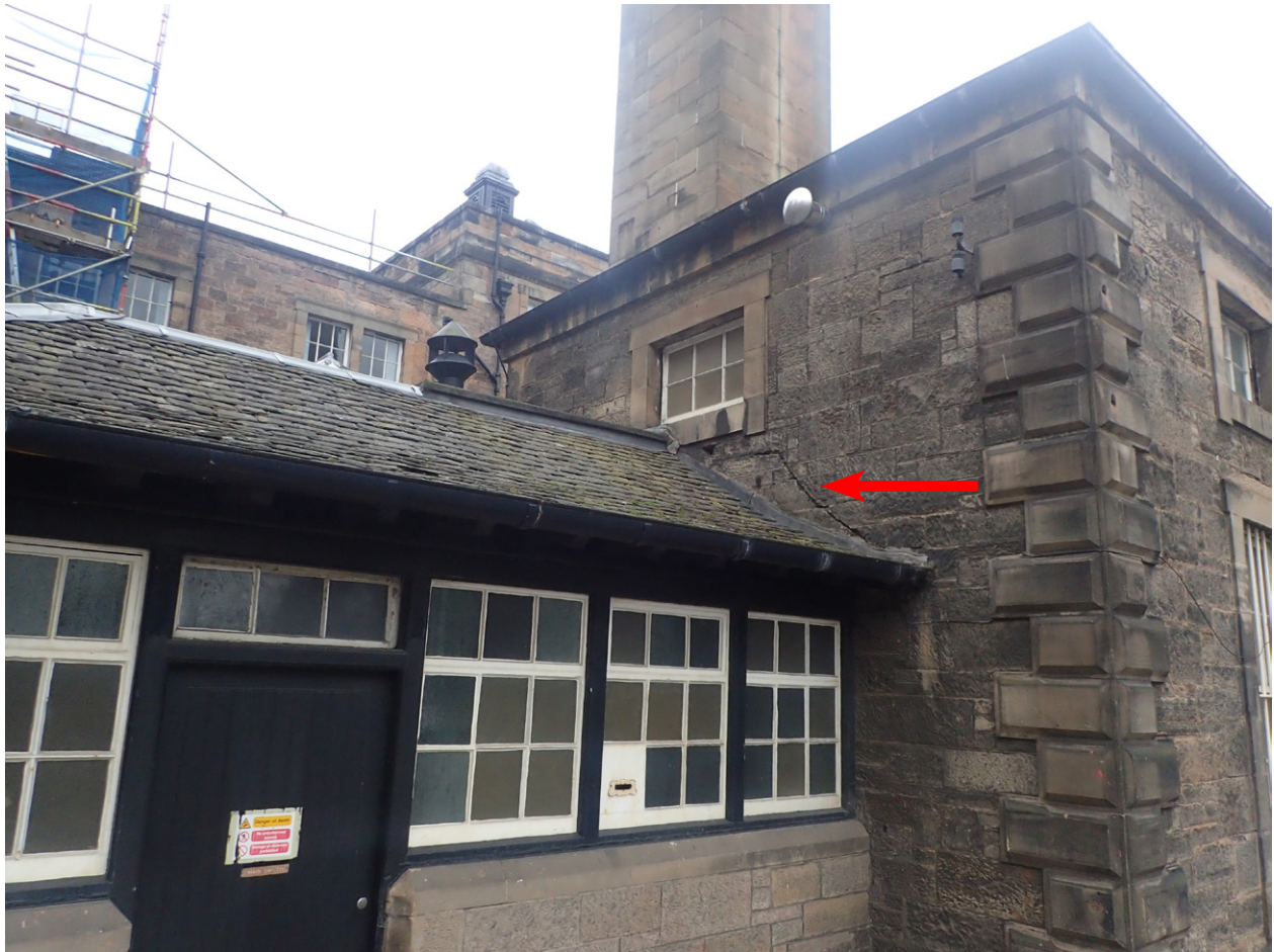
Fig. 15 - Exterior east-facing elevation showing the position of an earlier roofline
