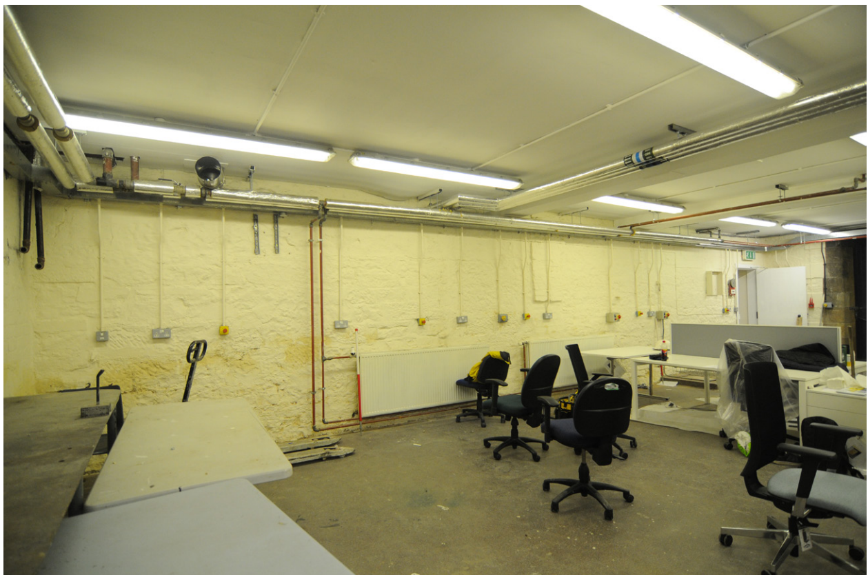
Fig. 10 - Ground floor Unit 3 workshop/storage general view
