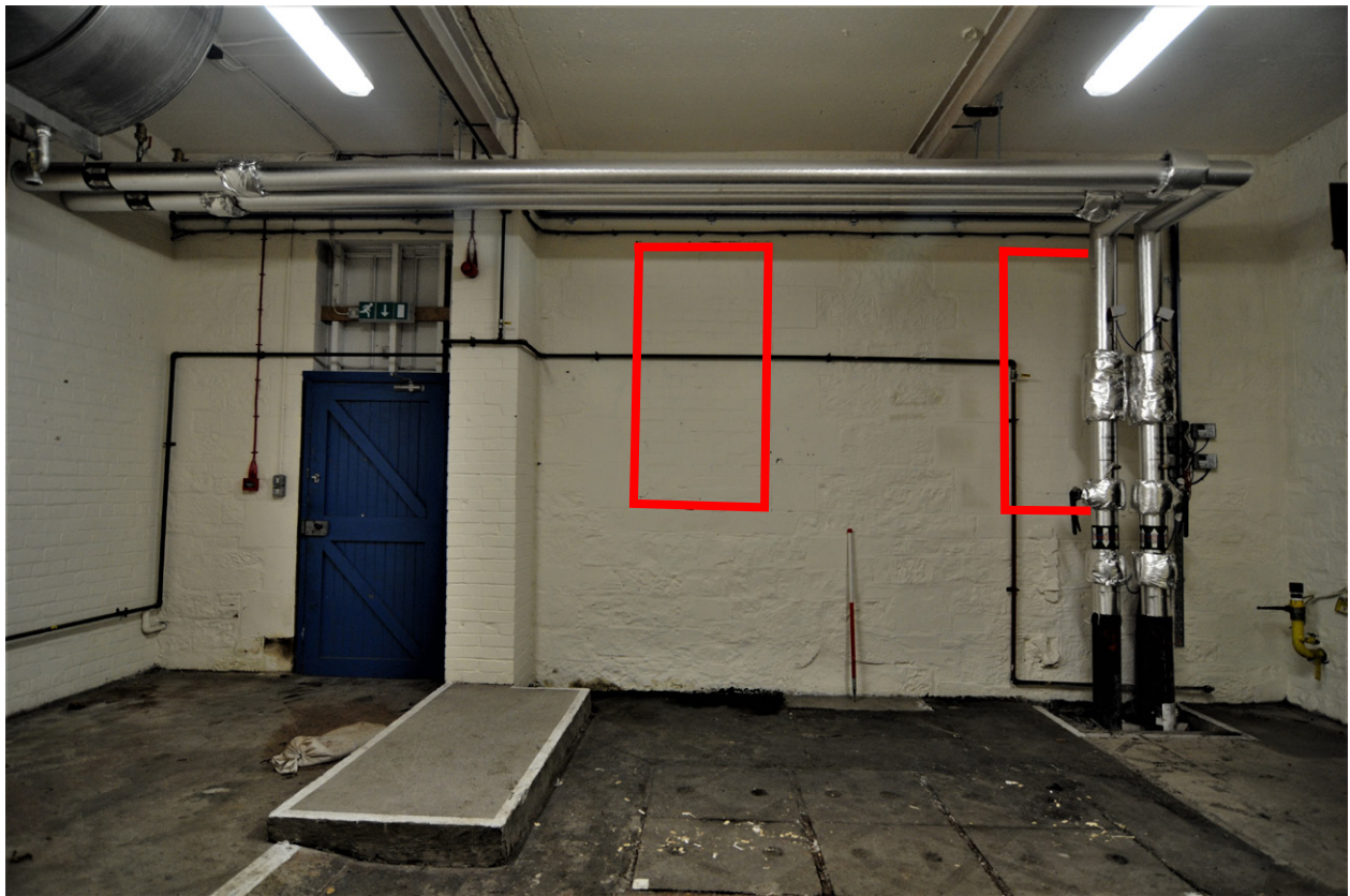
Fig. 9 - Ground floor Unit 1 workshop/storage showing two brick-blocked windows
