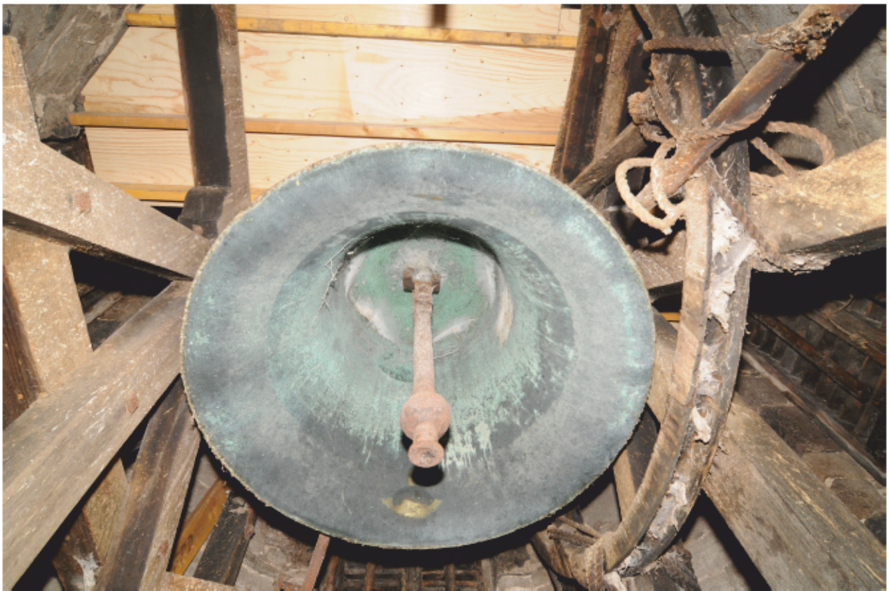
Fig. 33 - The church bell housed within its bell-frame
