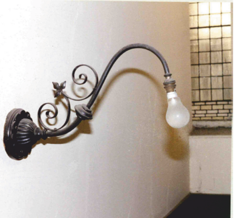
Fig. 34 - A historical photograph of one of the electric stair lights © Culture Perth and Kinross
