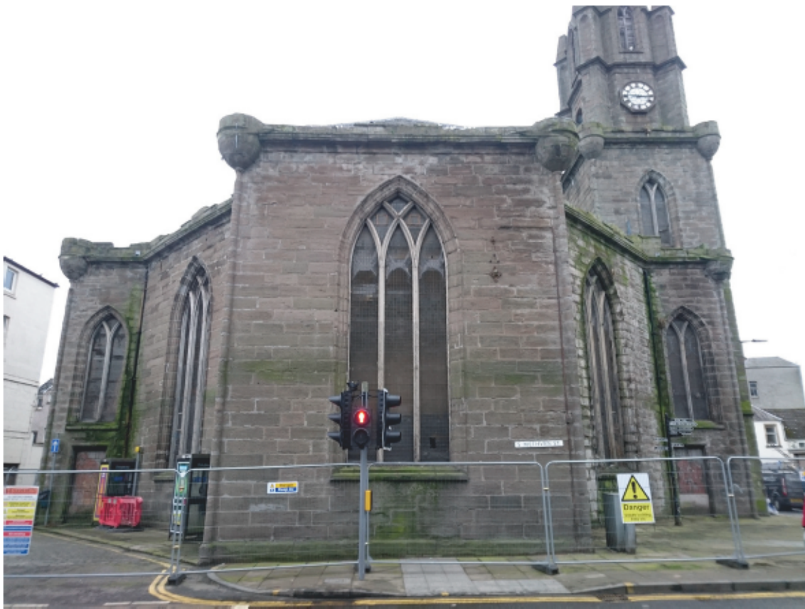
Fig. 5 - General view of the east-facing elevation before the scaffold was erected
