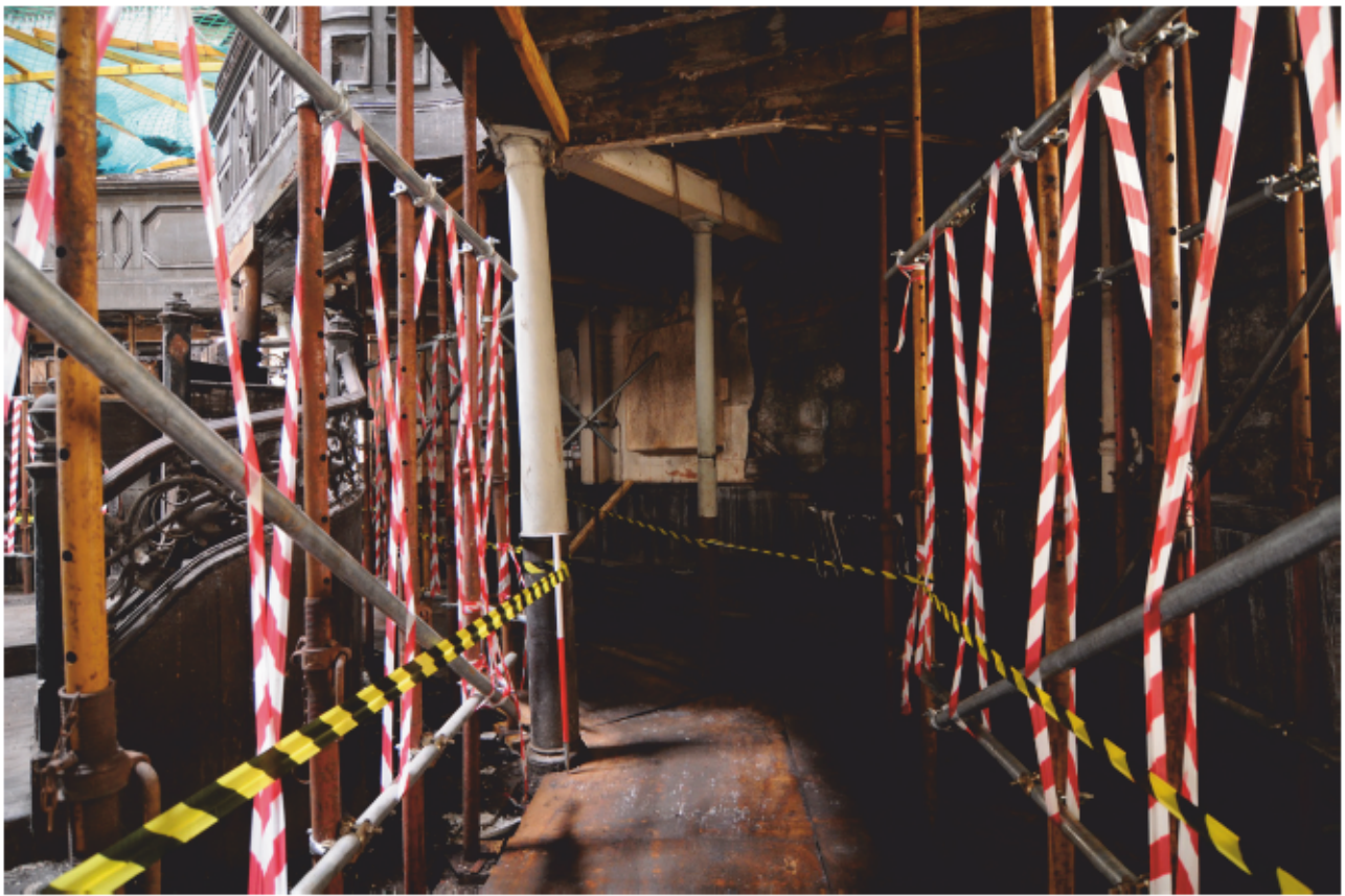
Fig. 13 - Interior shot of two of the pillars supporting the gallery floor
