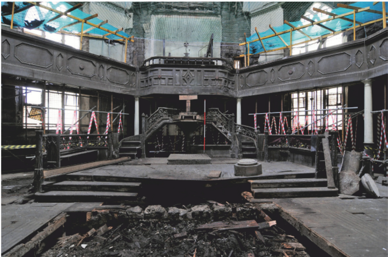
Fig. 10 - Interior south-facing elevation, with the remains of the pulpit
