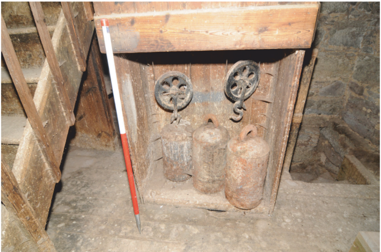
Fig. 30 - The clock weights housed in their weight chamber
