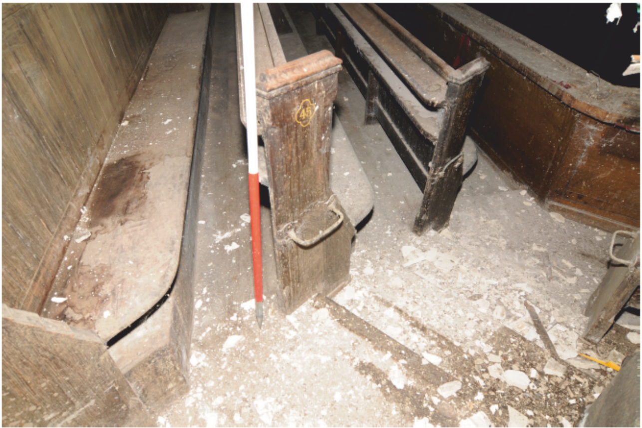
Fig. 27 - The hinged folding metal brackets on the end of the gallery pews
