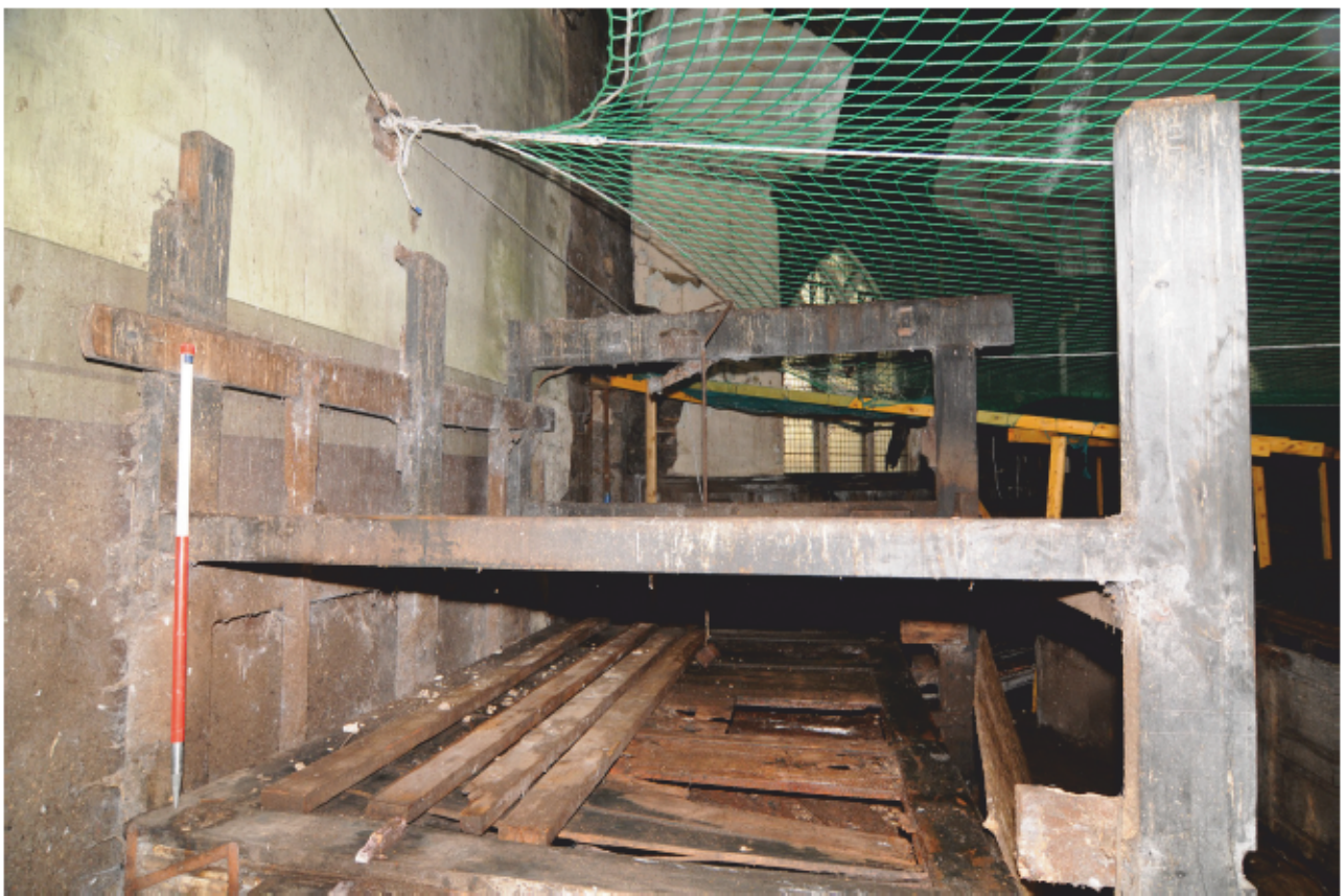
Fig. 25 - The remains of the organ frame situated on the north side of the gallery
