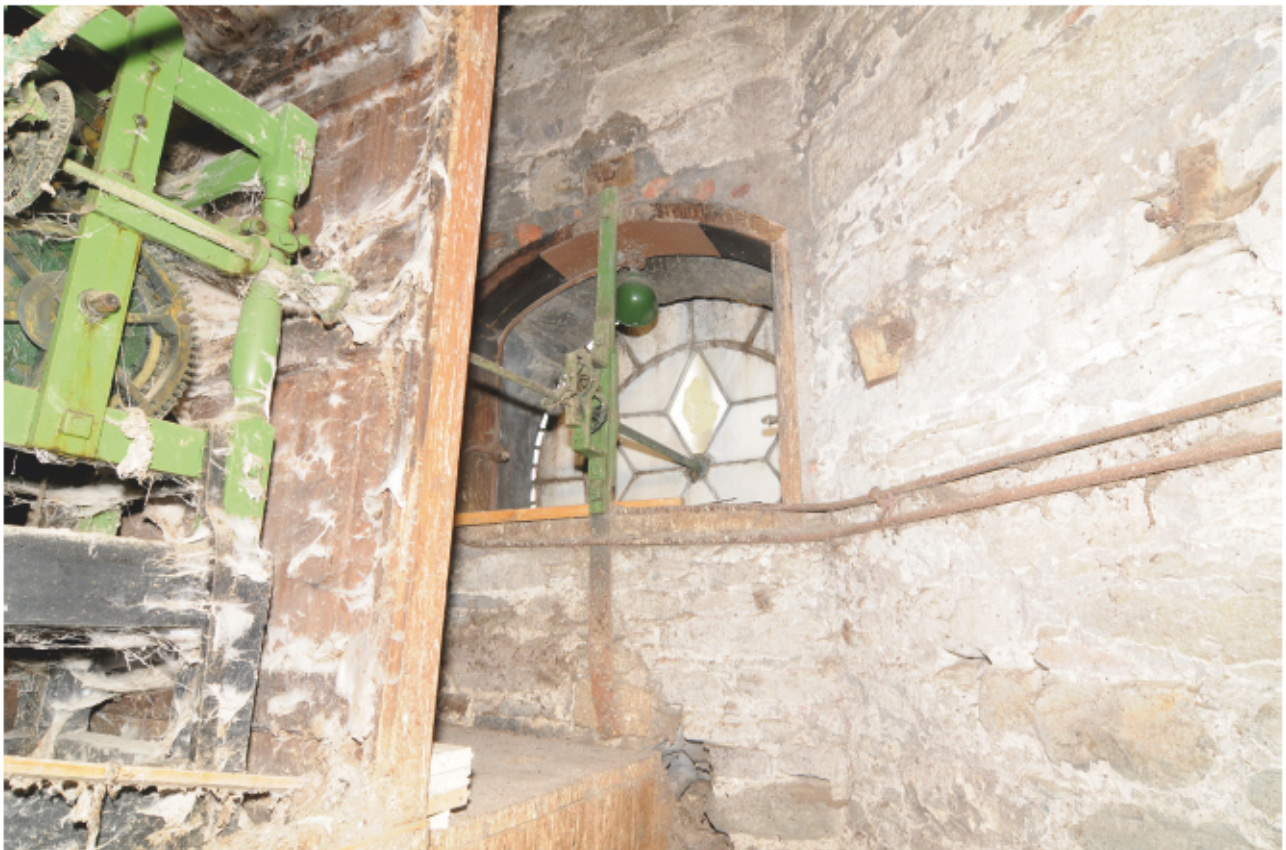
Fig. 32 - East-facing clock-face with turning mechanism and electric back-lighting lamp
