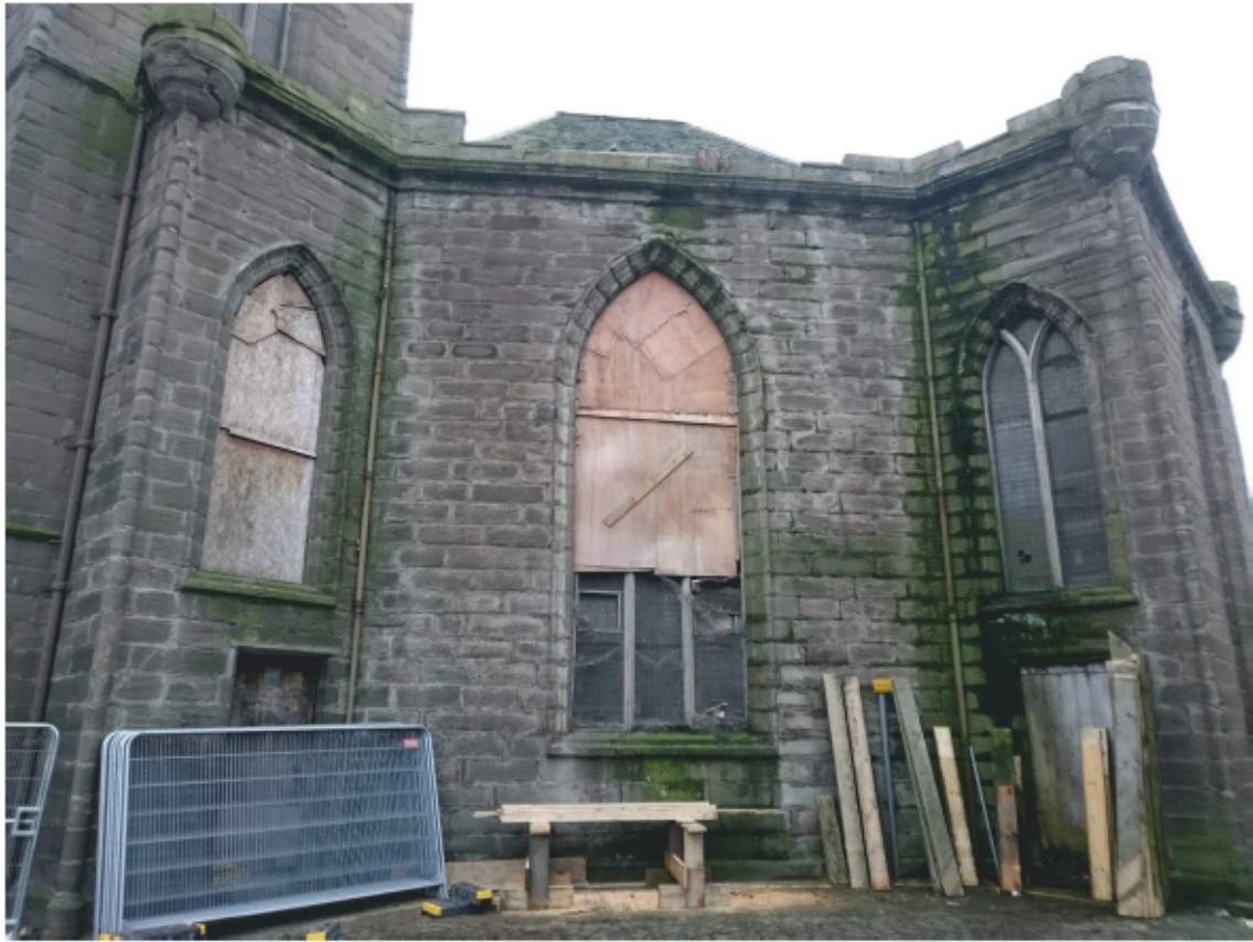
Fig. 7 - General view of the west-facing elevation before the scaffold was erected
