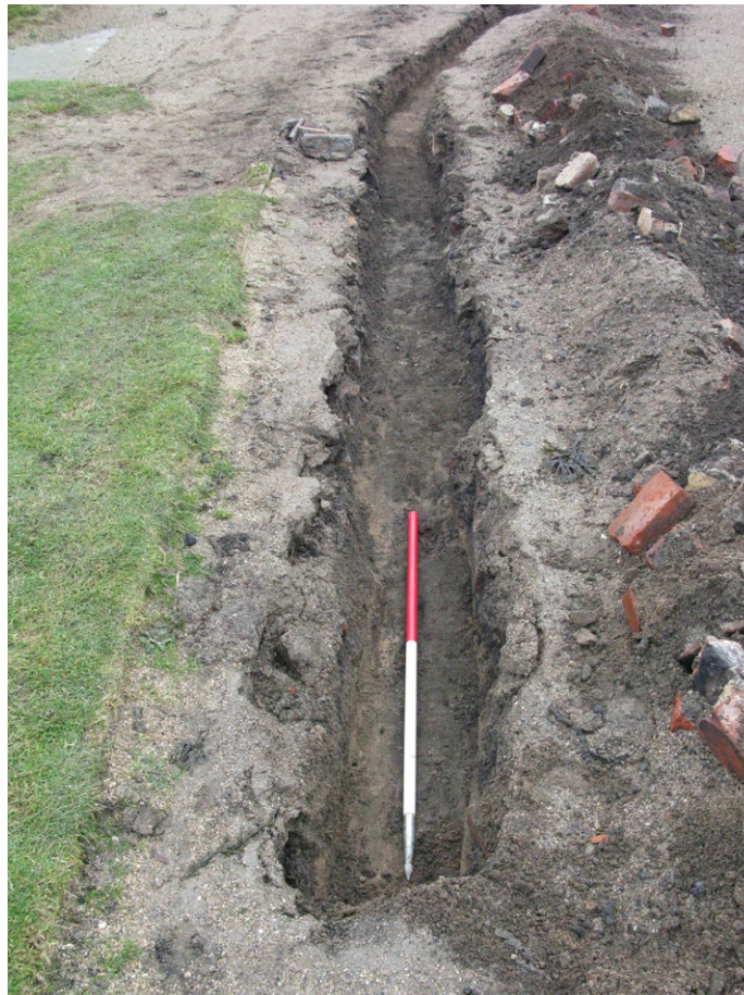
Fig. 7 - General view of trench
