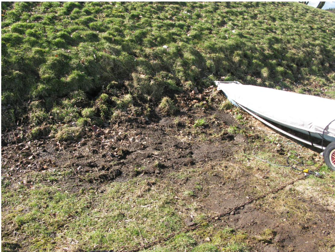
Fig.11 - Trench 4, post excavation and re turfing
