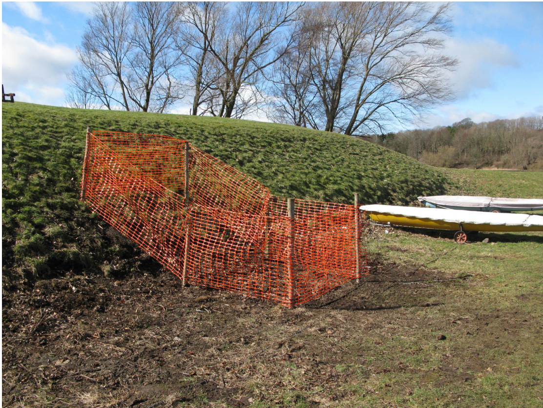
Fig. 10 - Trench 3, post excavation and netlon fencing
