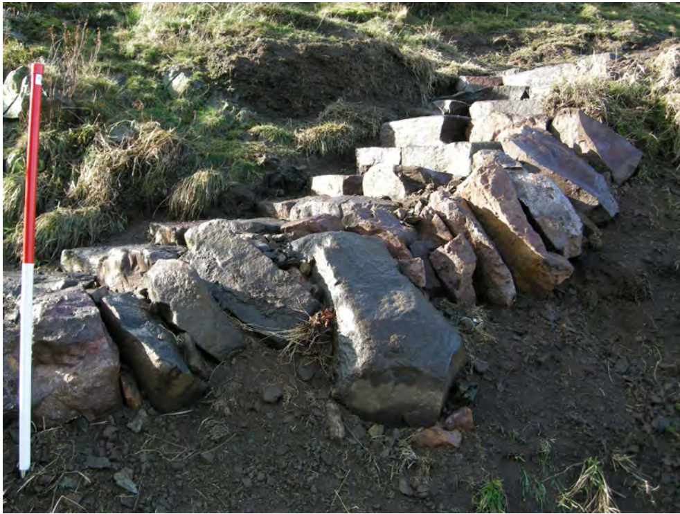
Fig. 6 - Completed stone revetment Area 1
