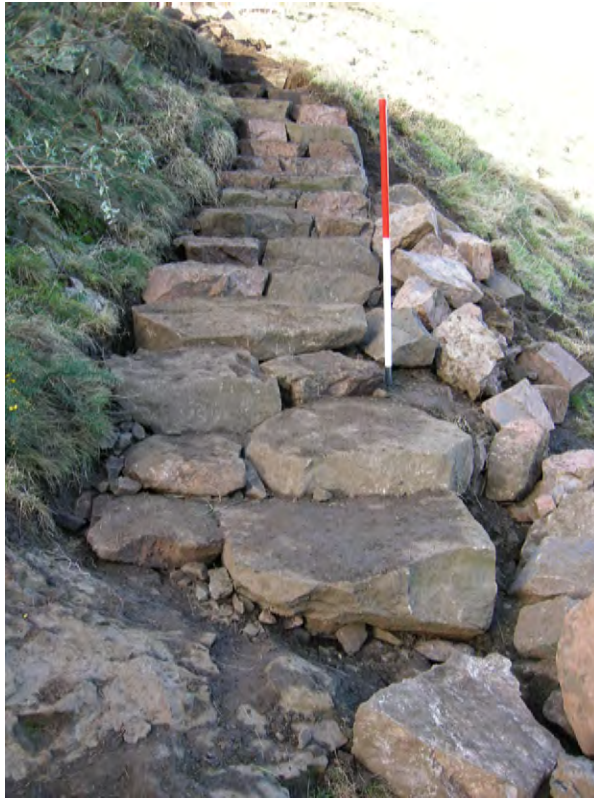
Fig. 2 - Detail of finished pitching in Area 1
