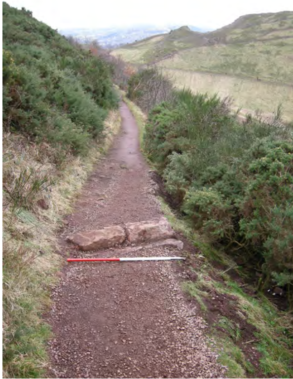
Fig. 12 - Completed waterbar and surfacing Area 3
