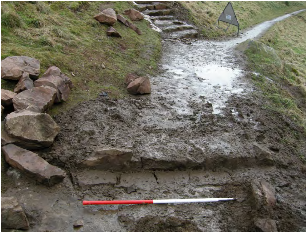
Fig. 8 - Join between Area 1 and 2
