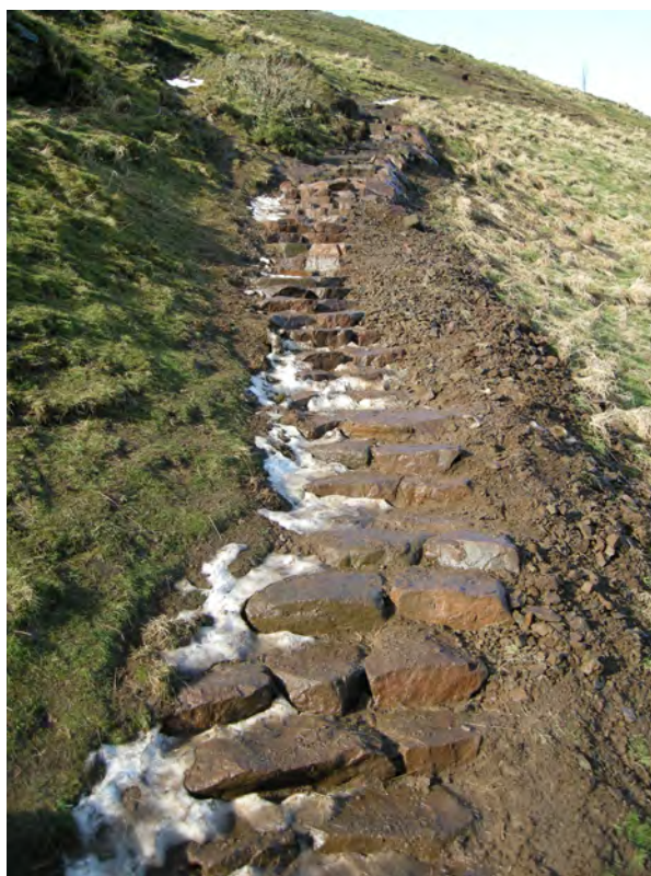
Fig. 5 - Completed pitching Area 1
