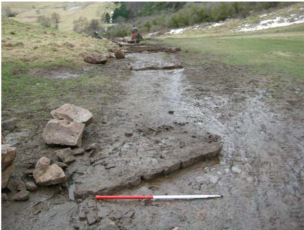
Fig. 7 - Working shot and completed waterbars Area 2
