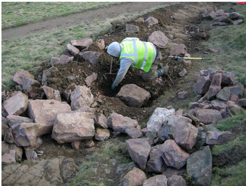
Fig. 4 - Working shot Area 1
