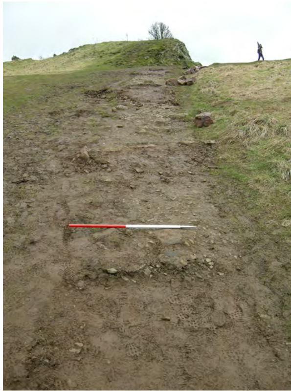
Fig. 10 - Completed waterbars Area 2
