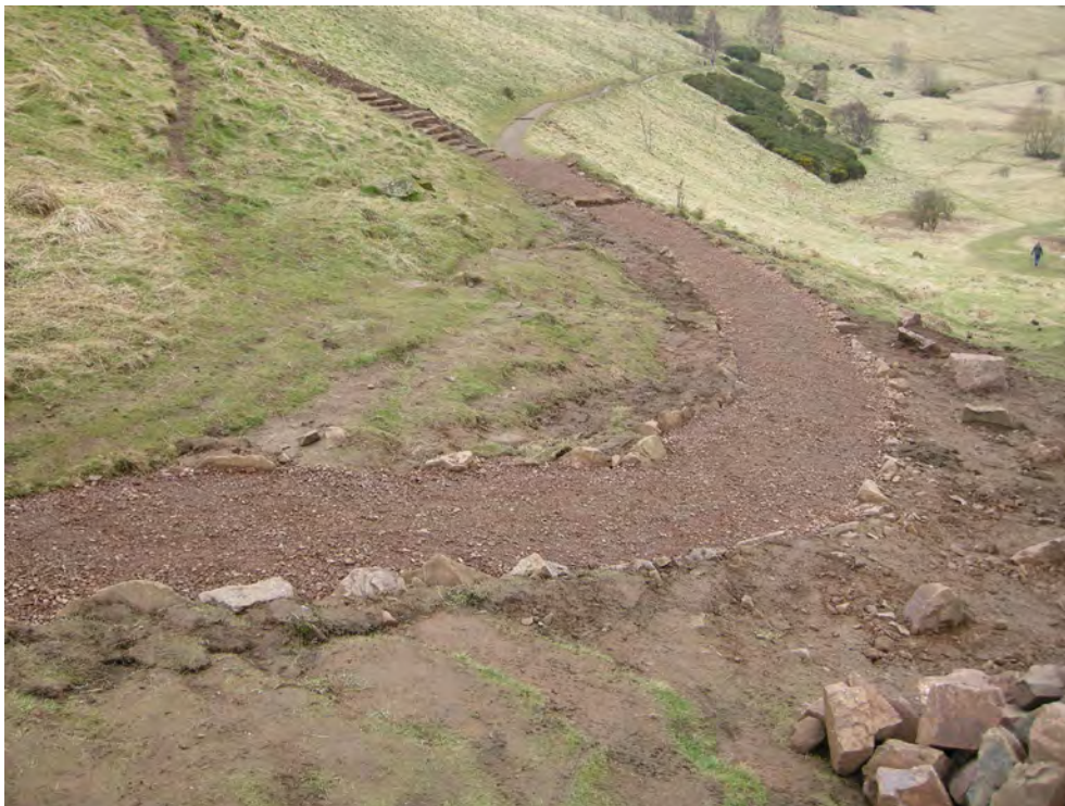
Fig. 9 - Completed path surfacing Area 2
