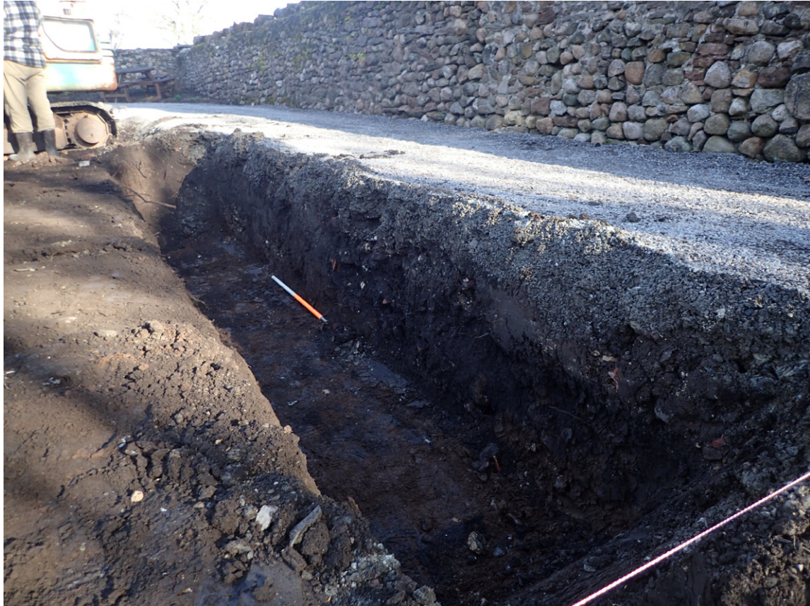
Fig. 4 - Example of the foundation trenches
