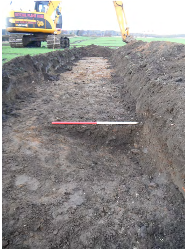
Fig. 15 - Trench 67, Feature 6701 (015) SE facing section
