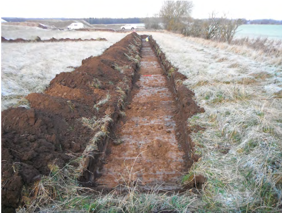
Fig. 4 - Trench 2 general view from the SSE
