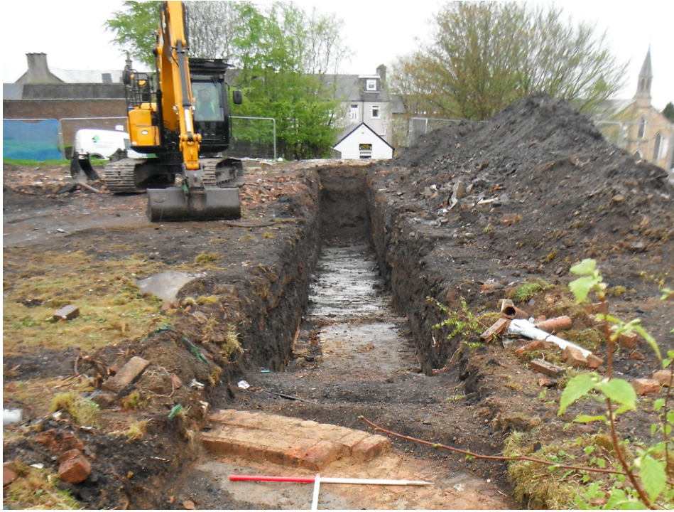
Fig. 4 - Trench 1 excavated from the North-West with wall 101 in the foreground
