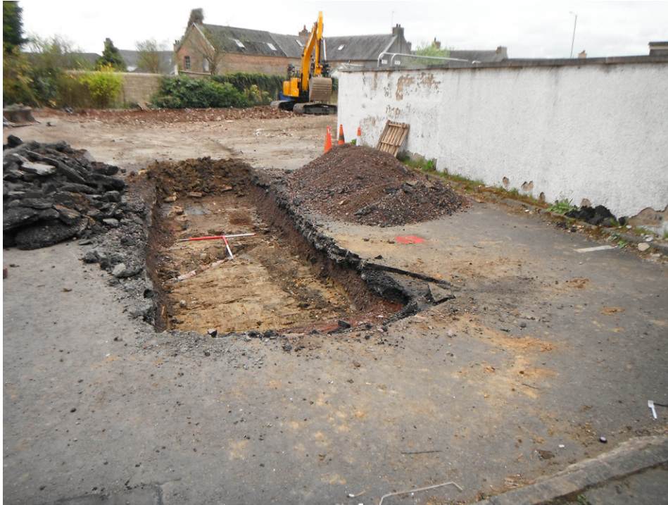
Fig. 12 - Trench 7 and the northern part of the site at 11 Kirkton Street from the NNE
