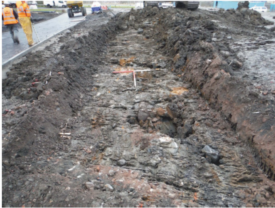
Fig. 5 - General shot showing nature of soil deposits
