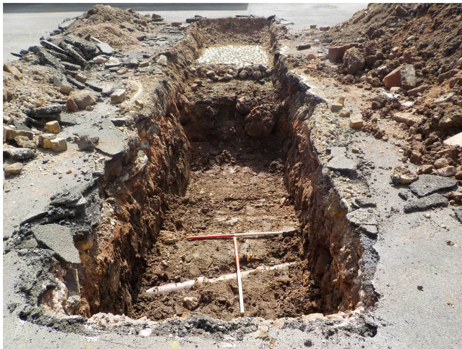
Fig. 3.2 - Trench 2, facing south-east
