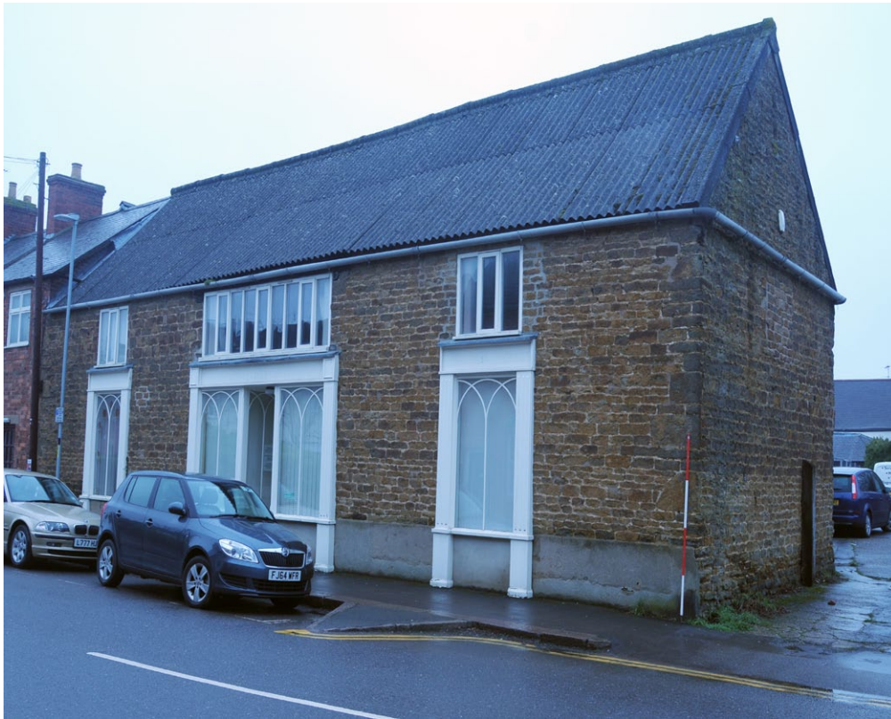
Fig. 9a - Front elevation, Unit 1, facing NW
