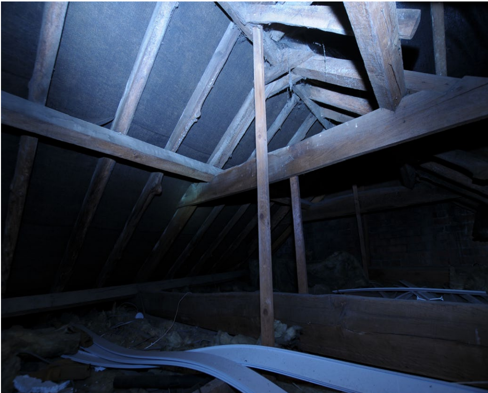
Fig. 9p - Shot of Attic, Unit 2, facing SW
