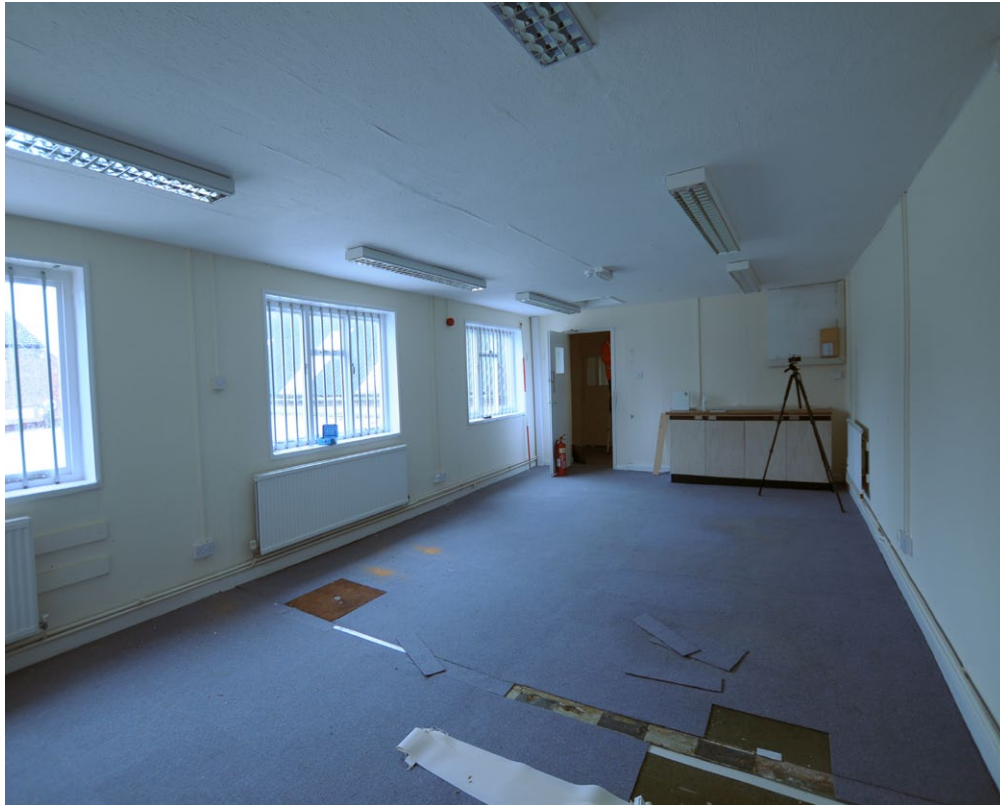
Fig. 9s - 1st floor office, Unit 4, facing SE
