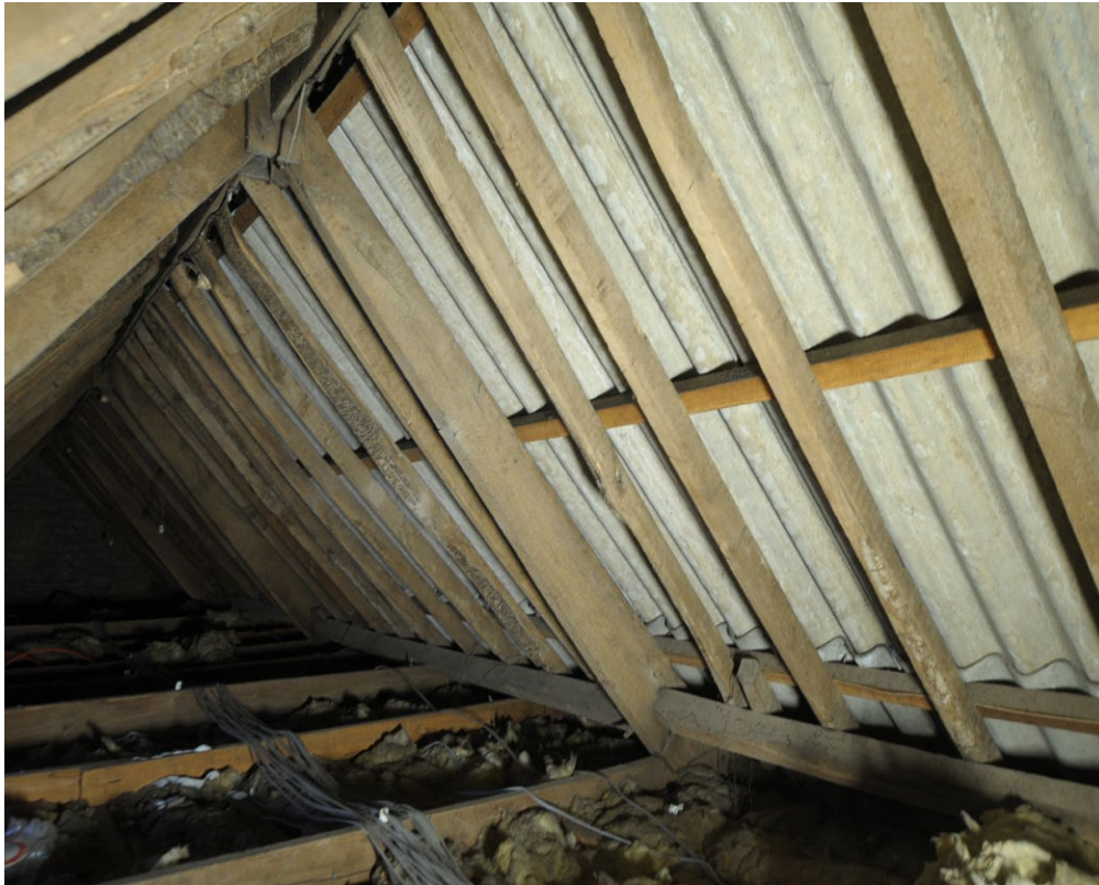
Fig. 9i - Photo of truss, Unit 1, facing SE
