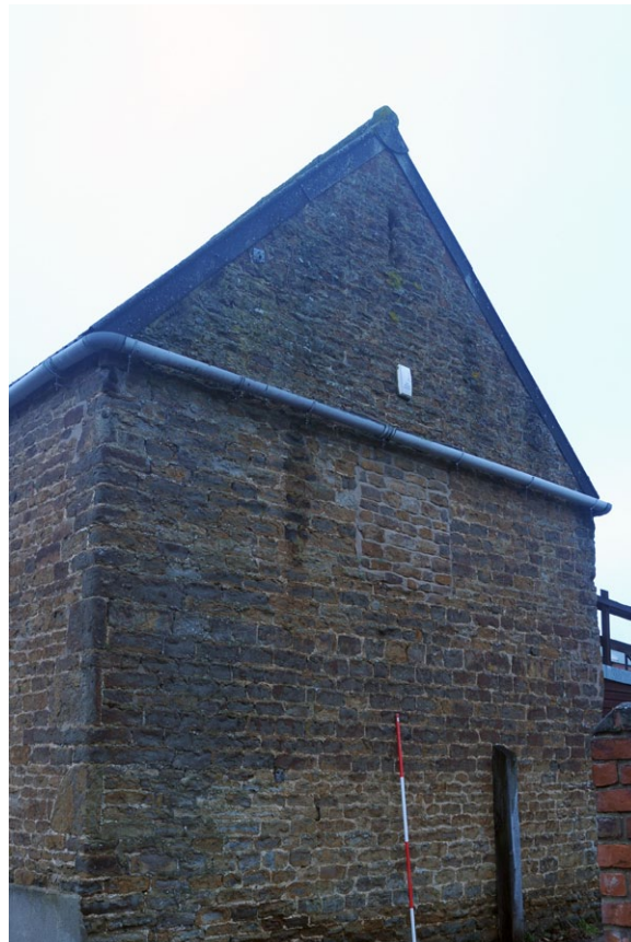
Fig. 9d - The E gable, Unit 1, facing NW
