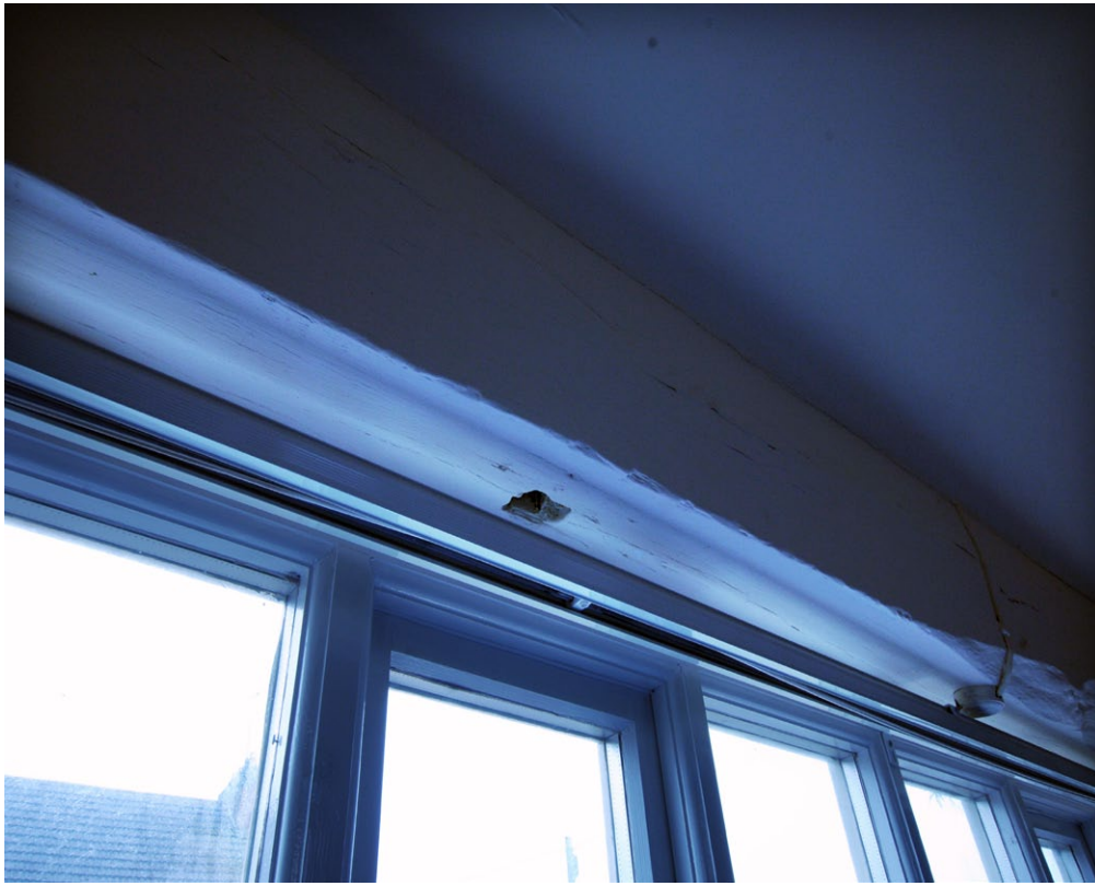
Fig. 9c - Beam across central window of Unit 1, facing SW
