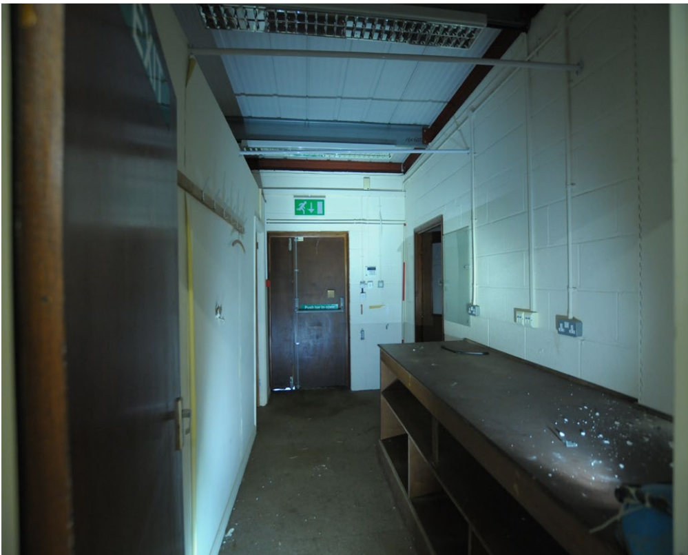
Fig. 9v - Central corridor, Unit 5, facing S
