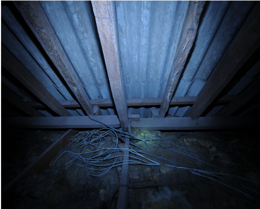
Fig. 9k - Detail of pegged purlin, Unit 1
