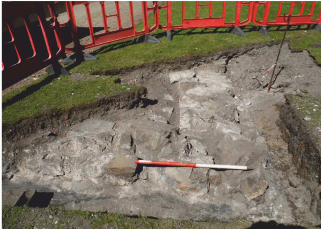
Fig. 4 - Foundations 004 and 005 from south
