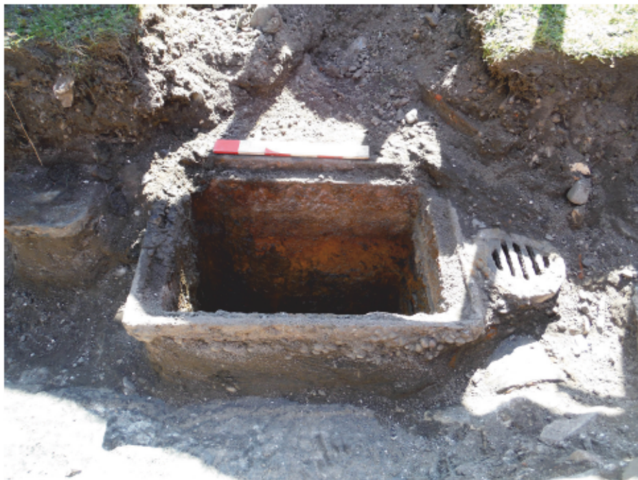
Fig. 5 - Drainage 006 from south
