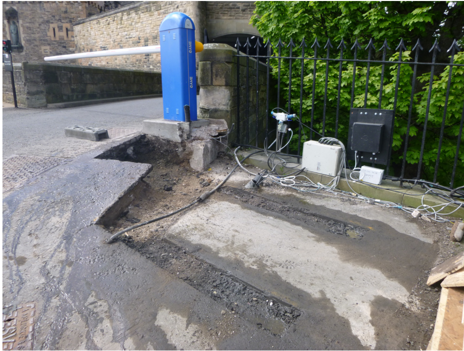
Fig.2 - Post-ex view of ground breaking works.
