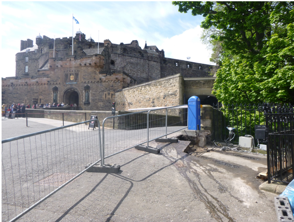
Fig. 3 - General view of location of works
