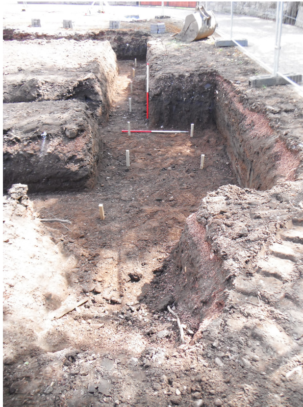
Fig. 4 - Wider foundation trench for entranceway to the south-west
