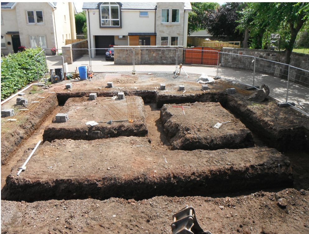
Fig. 3 - Post-excitation view of the south-eastern foundation trenches
