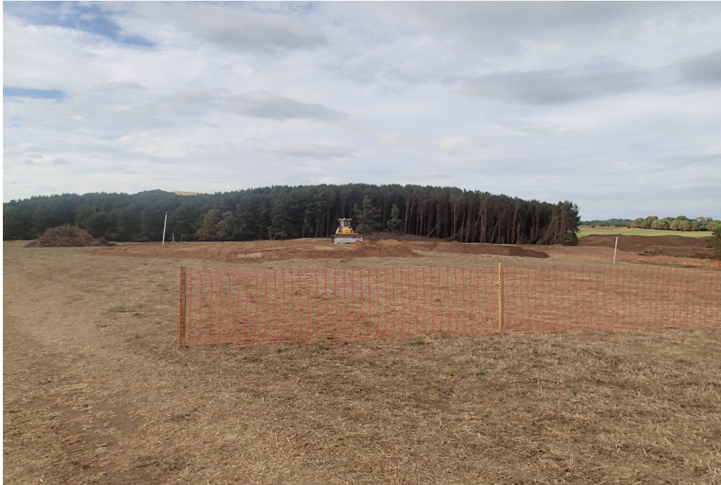
Fig. 4 - Working shot showing demarcation fence and practice tee platform, facing north
