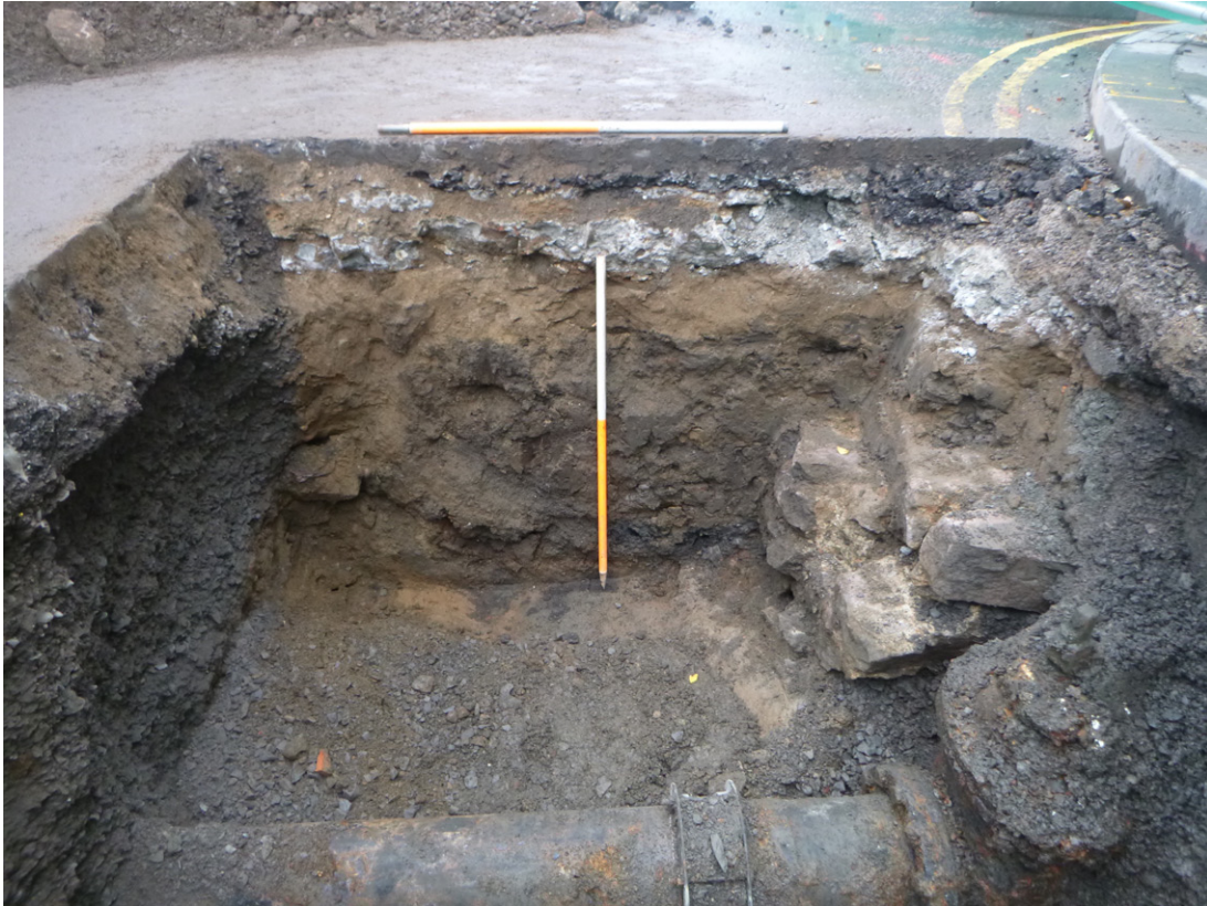
Fig. 2 - West-facing section of Trench 1 showing surviving deposits
