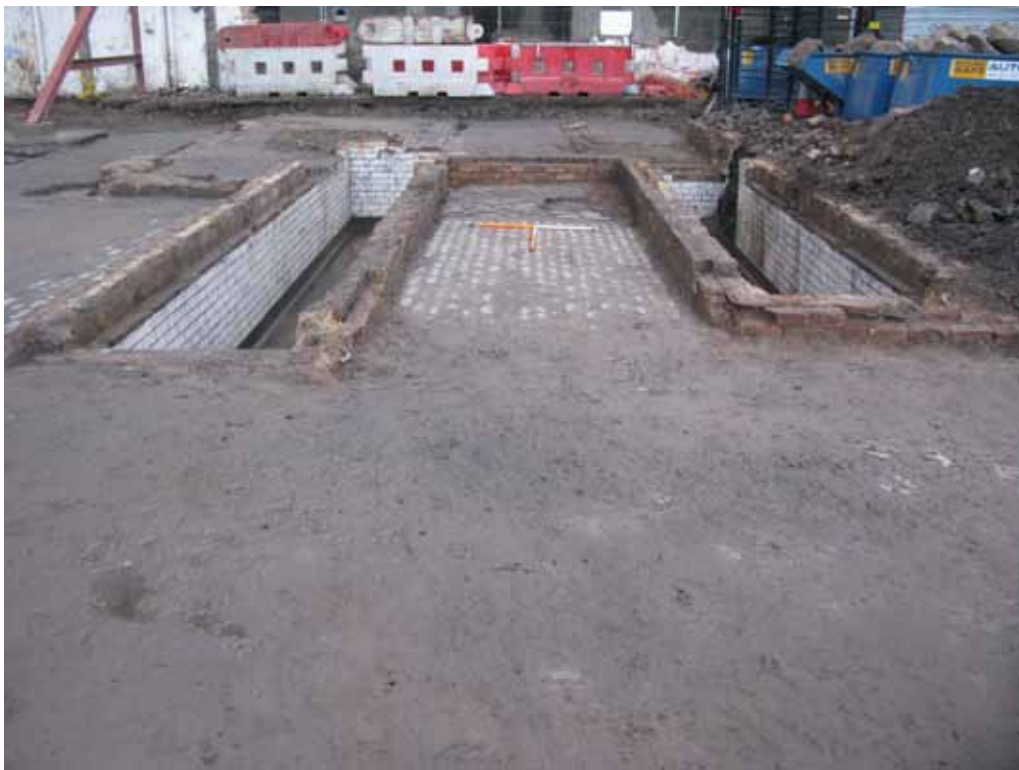
Fig. 14 - Southern half of mechanic inspection pit 285
