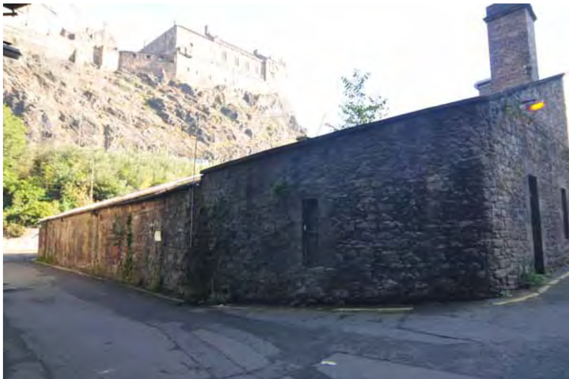
Fig. 6 - Western and southern boundary wall of Area 1
