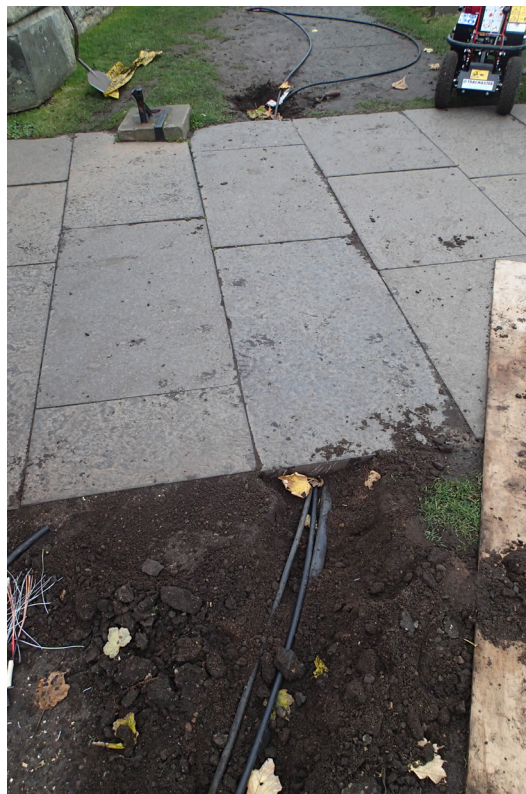
Fig. 3 - Cable being pulled beneath slabs at W entrance
