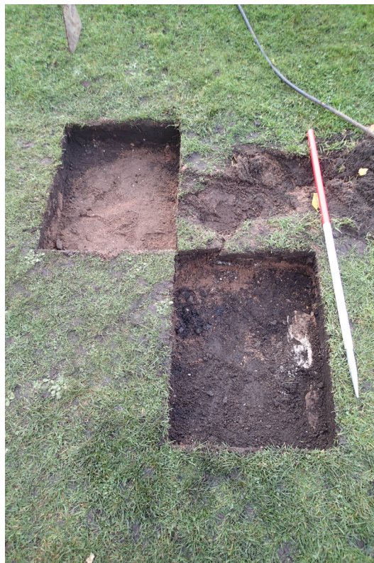
Fig. 5 - Plinths for lights 1 and 2 at SW corner of Cathedral
