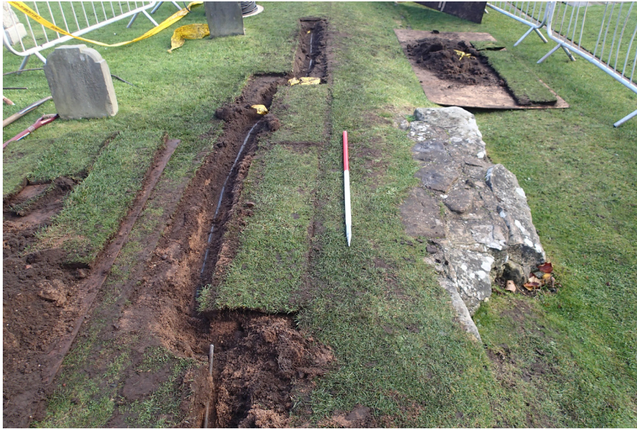
Fig. 4 - Cable trench being diverted around foundations at north side of Cathedral
