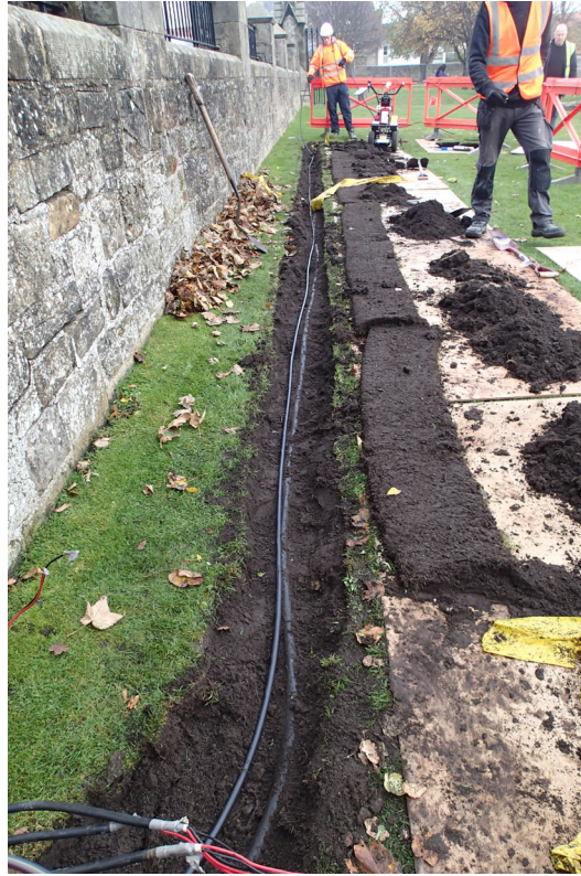
Fig. 2 - General shot of cable trench along the western boundary wall
