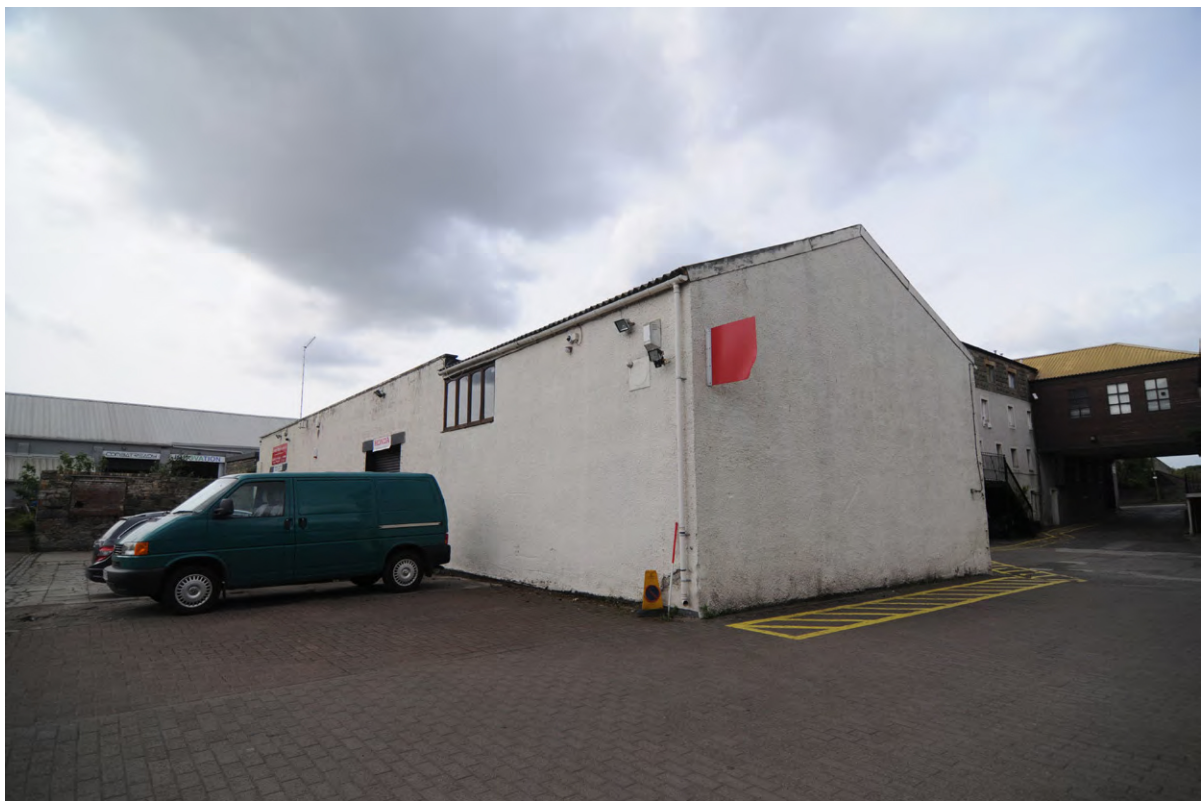
Fig.14 Building J, north-facing gable and east-facing elevation
