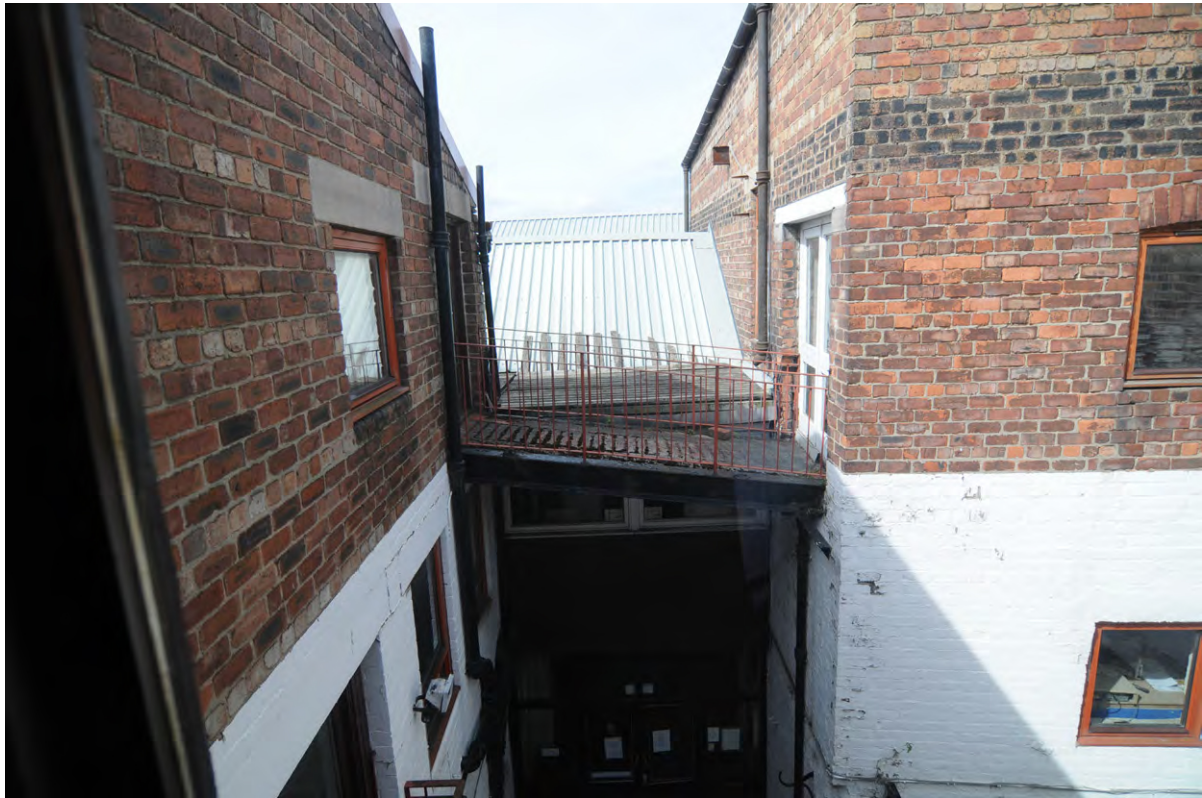
Fig.11 Building G behind a first floor gantry
