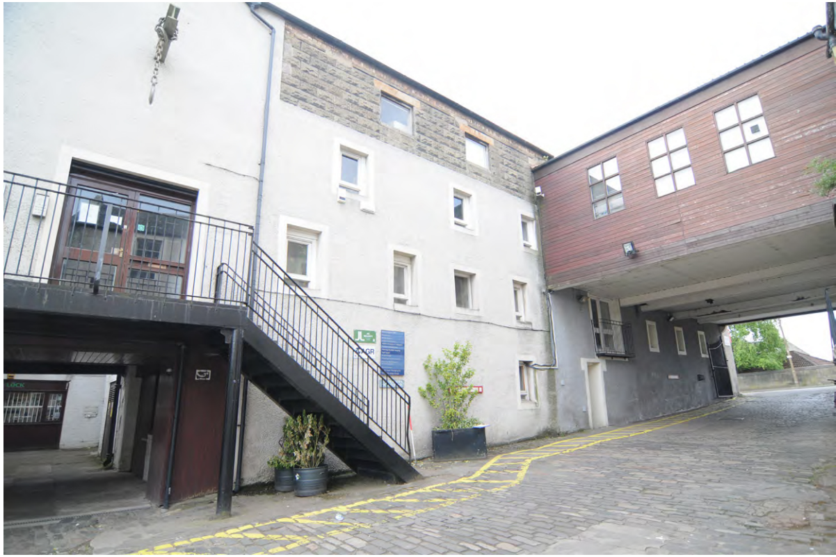
Fig.7 Building D, north-facing elevation with connecting Building C
