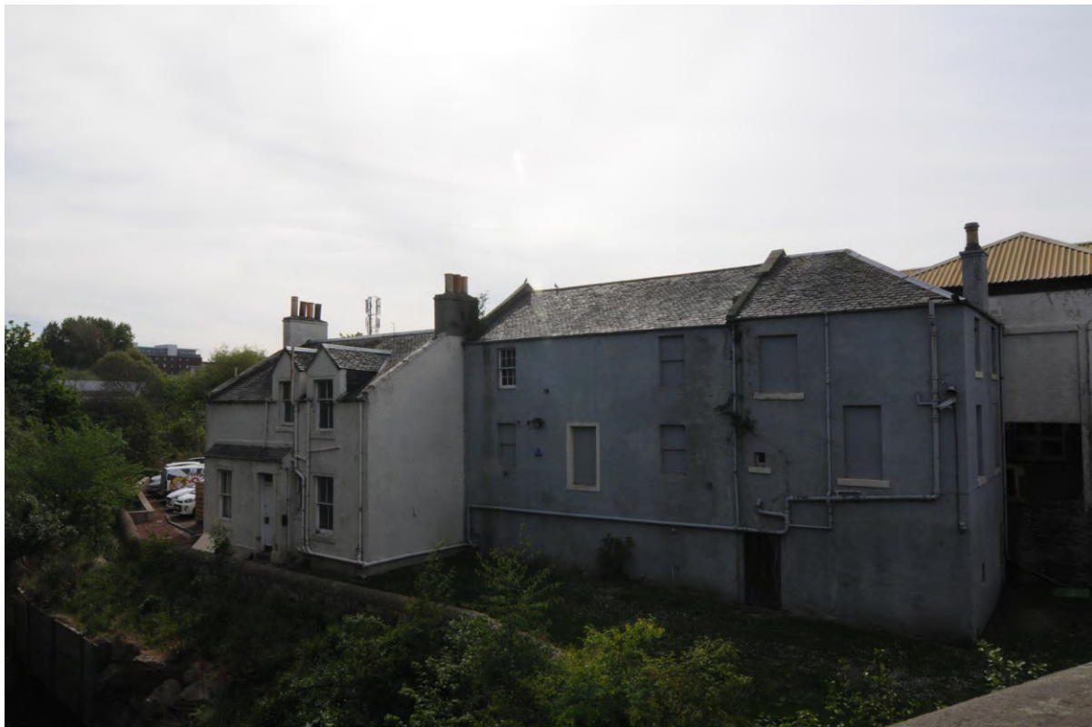
Fig.3 Building A, North-facing elevation with pitched and hipped roofline
