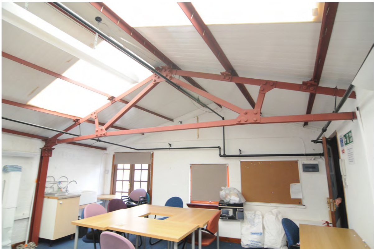
Fig.12 Building H interior composite steel roof truss
