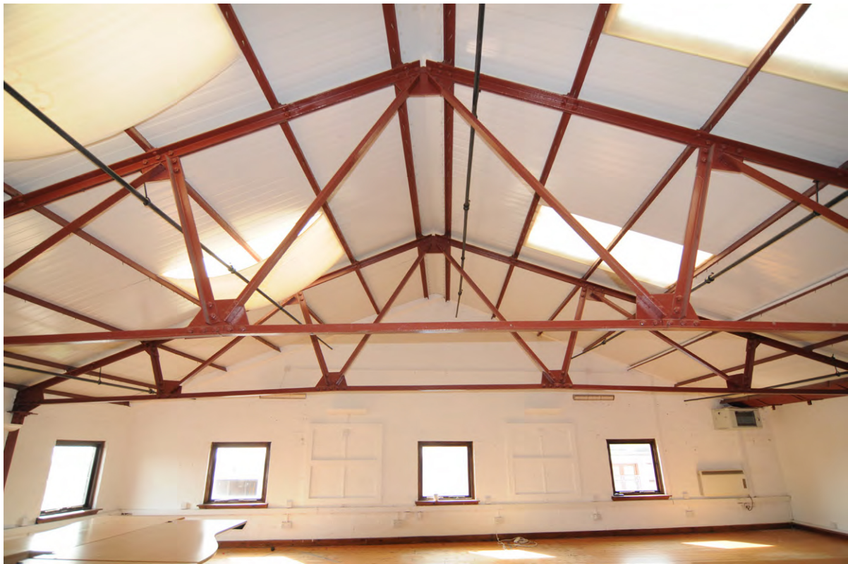
Fig.13 Building I, interior composite steel truss
