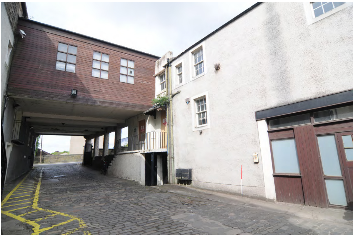
Fig.6 Building C supported by pillars and underpass
