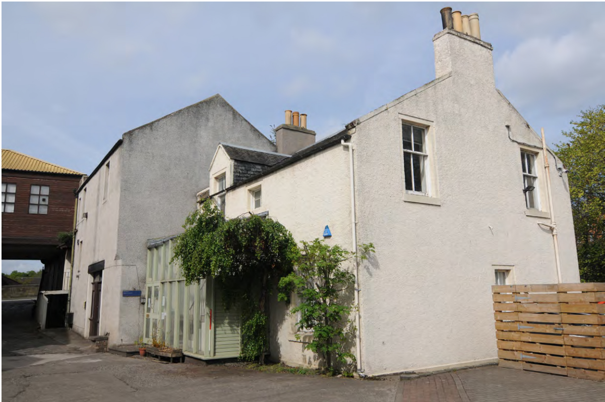
Fig.5 Building B, south and east-facing elevations
