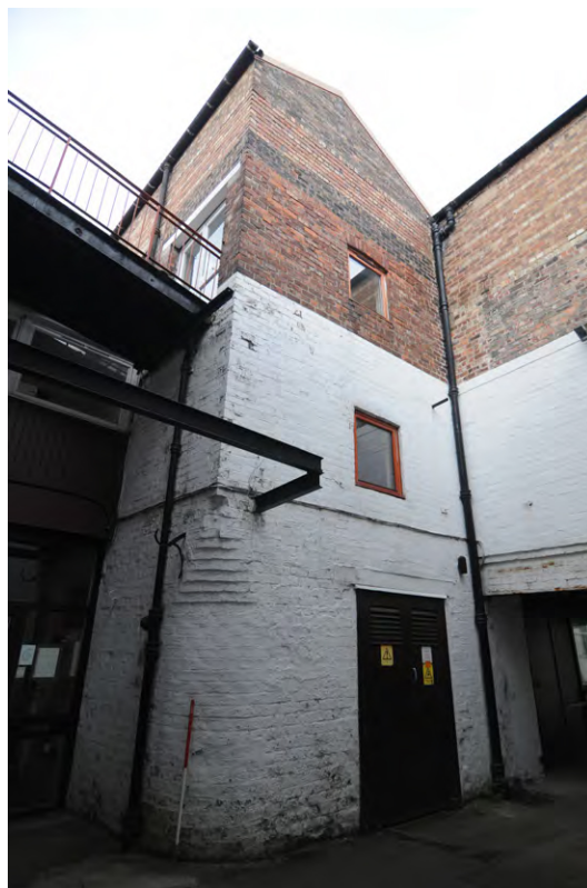
Fig.10 Building F, brick-built gable within the courtyard
