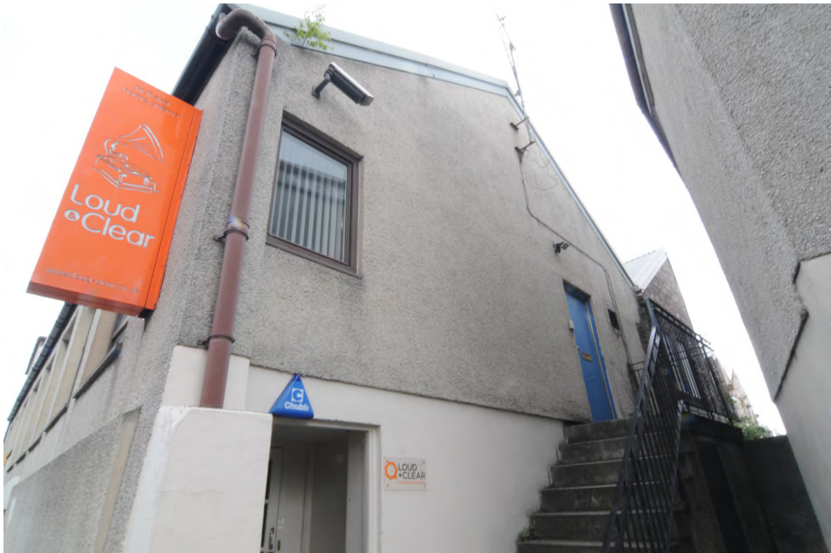
Fig.9 Building E south-facing gable walls
