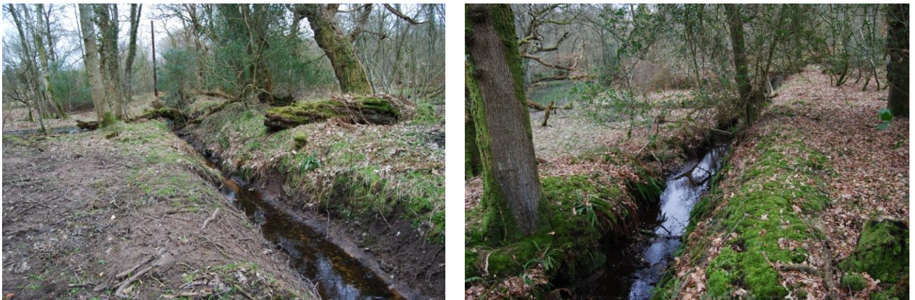
Illus 44 L: looking north along the west bank, with secondary woodland on LHS. R: internal ditch running north east (PQ C105, 113)
