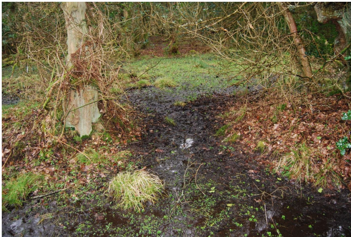
Illus 20 There are several cross drains like this one, on the west bank of Cpt E (PQ C346)
