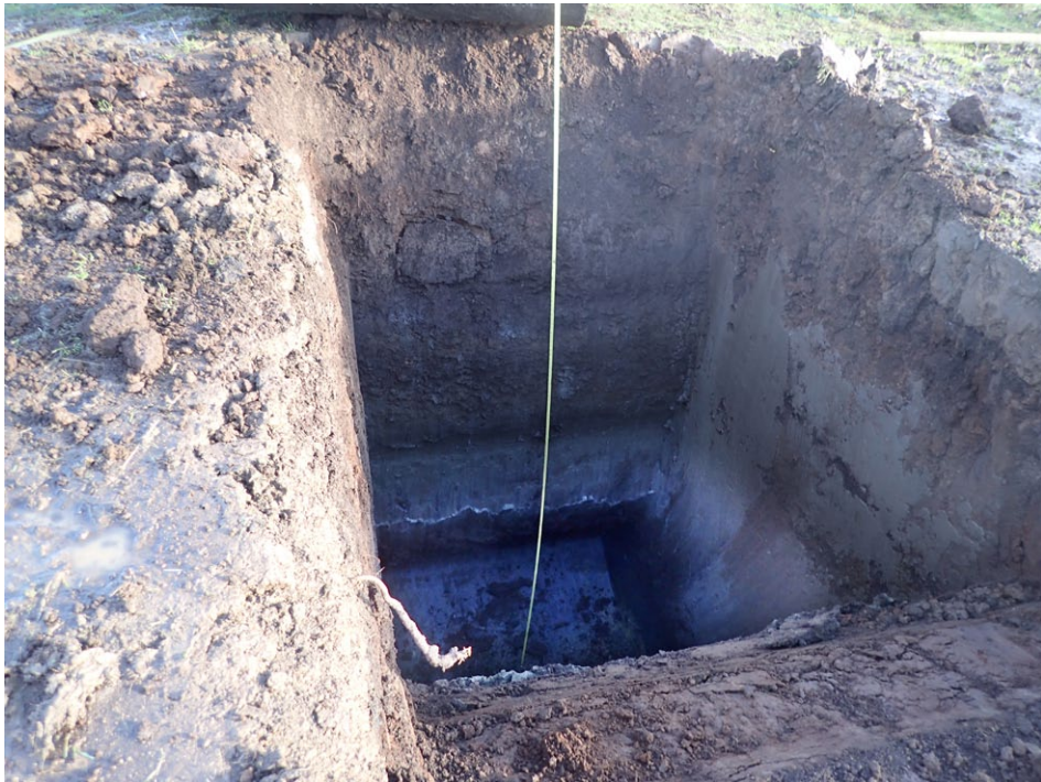
Fig. 17 - Eastern sondage, Trench 4 (SS3), looking E
