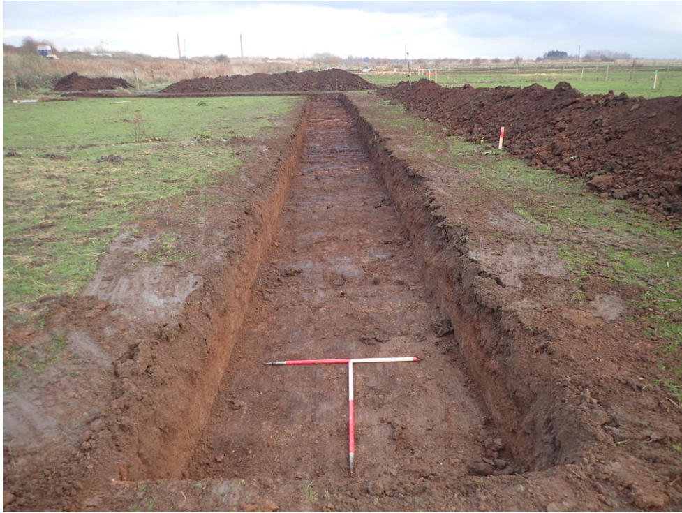
Fig. 14 - Trench 3, looking E
