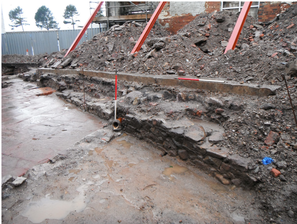
Fig. 10 - Wall 025 abutting dye works wall 024 from the NE
