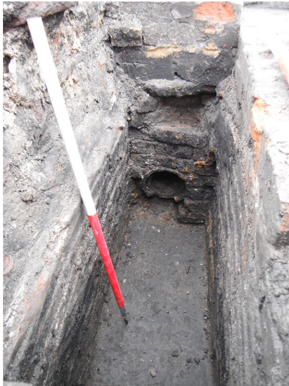
Fig. 23 - Pipe 035 in the base of feature 032 from the WNW
