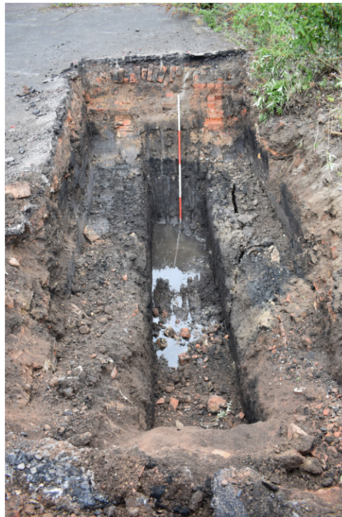
Fig. 3.2 - General view of trench 2, looking east
