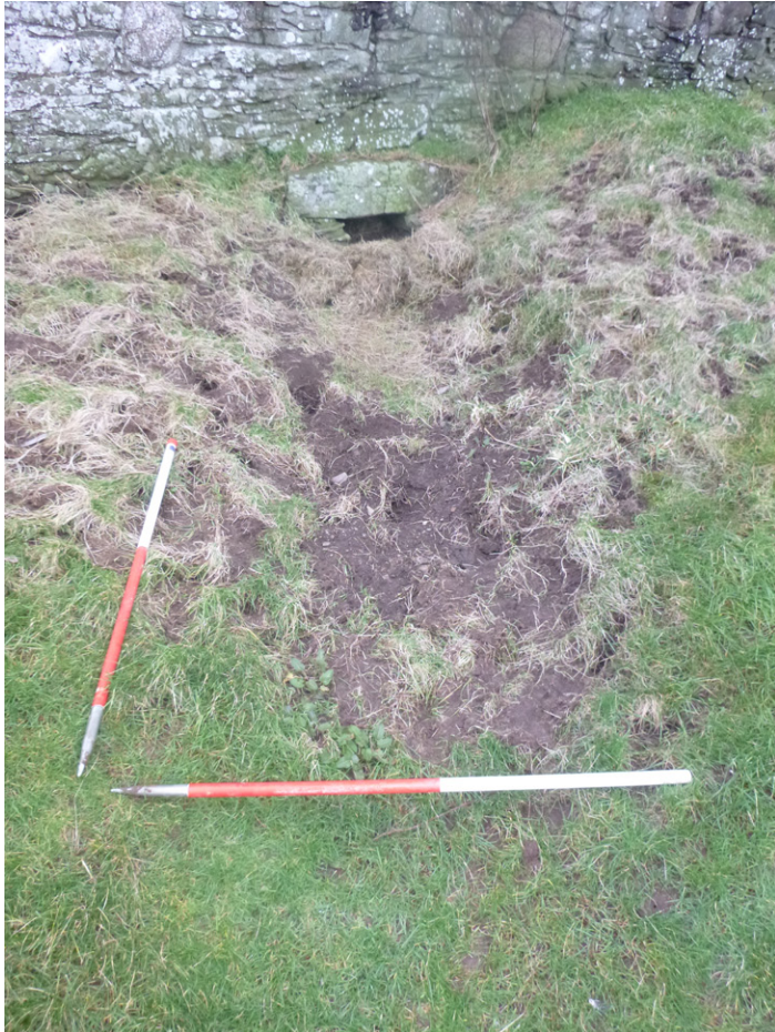
Fig. 8: Badger burrow and scrape damage at western wall of tower
